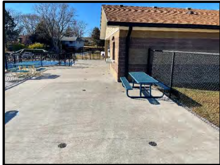
Picture 4: Floor Drains – 11/21/2023
