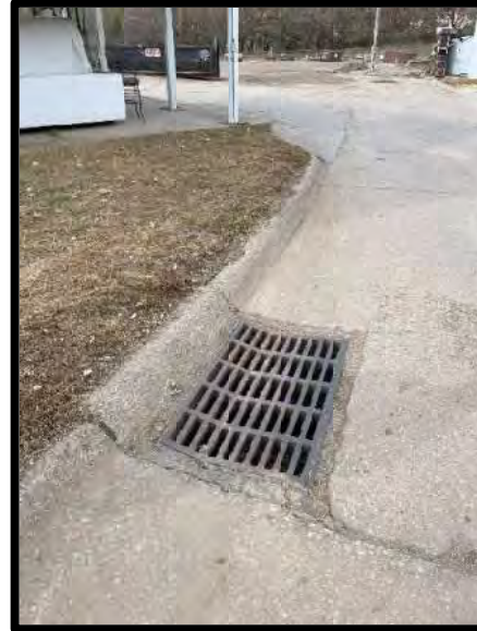
Picture 6: Inlet West of Sand/Gravel Storage – 11/14/2023
