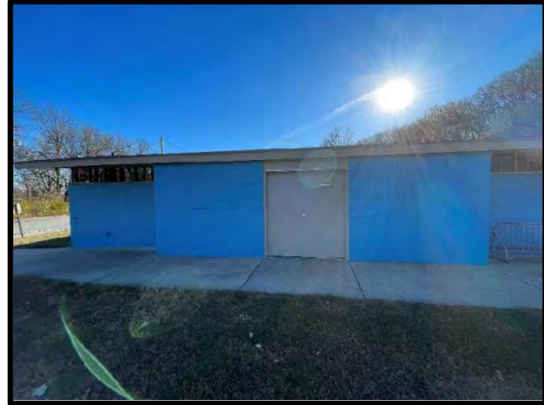
Picture 6: Main Facility Entrance – 11/21/2023
