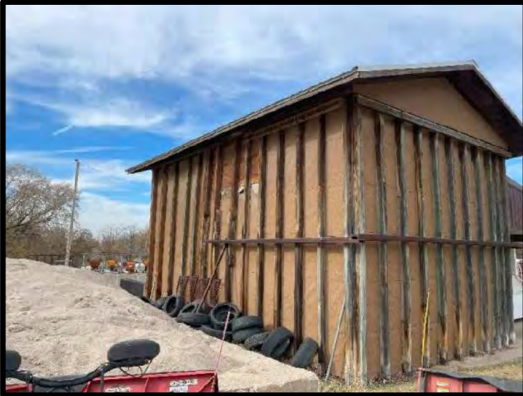
Picture 5: South and West Sides Salt Storage Building – 11/14/2023
