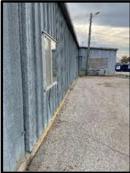
Picture 15: Downspouts on Street Department Storage Building – 11/16/2023
