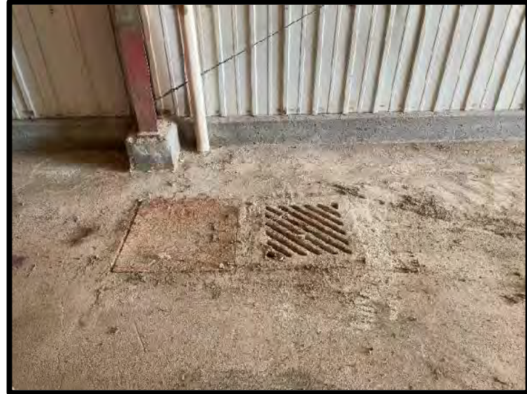
Picture 34: Indoor Drain Pit – 11/14/2023
