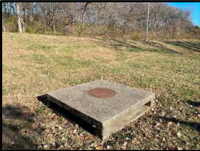
Picture 7: Area Inlet North of Facility – 11/21/2023
