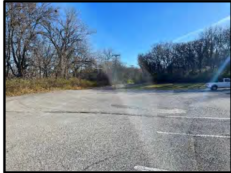
Picture 10: Parking Lot – 11/21/2023
