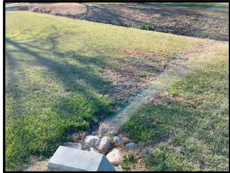
Picture 6: Pool Drainage North Outlet – 11/21/2023
