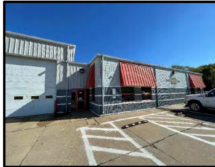
Picture 18: Exterior of Facility – 10/16/2023
