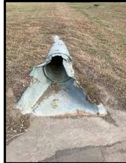
Picture 8: Flared End Section West of Salt Storage Building – 11/14/2023
