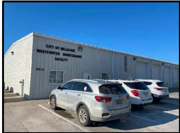
Picture 20: Main Office Building East Face – 11/28/2023
