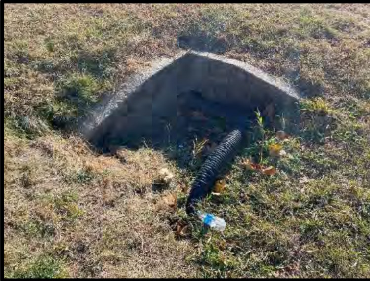
Picture 7: Culvert Inlet South of Pool – 11/21/2023
