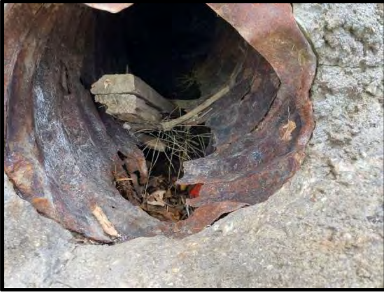
Picture 9: Culvert Drainage Pipe Invert – 9/14/2023
