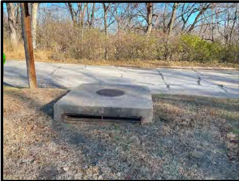
Picture 3: Area Inlet Southeast of Facility – 11/21/2023
