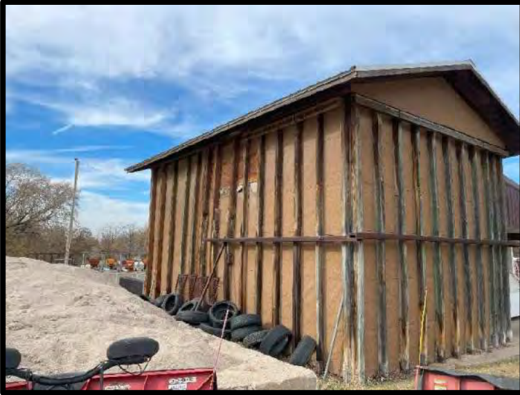
Picture 5: South and West Sides Salt Storage Building – 11/14/2023
