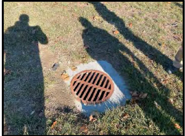
Picture 12: Area Inlet Southwest of Pool – 11/21/2023
