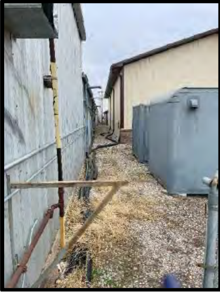
Picture 5: Downspout Extenders East Side Parks Storage Building – 11/16/2023
