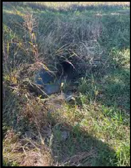
Picture 17: Culvert Inlet Southwest of Facility – 10/16/2023
