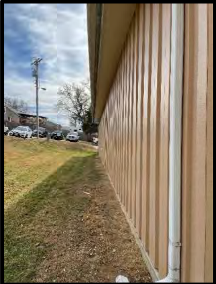
Picture 3: Downspouts on West side of Main Office Building – 11/14/2023
