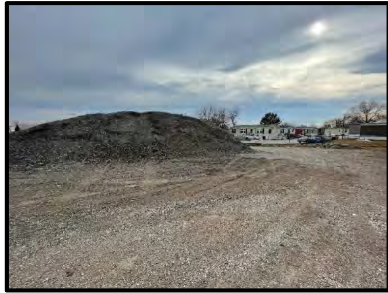
Picture 34: Asphalt Millings Stockpile – 11/16/2023
