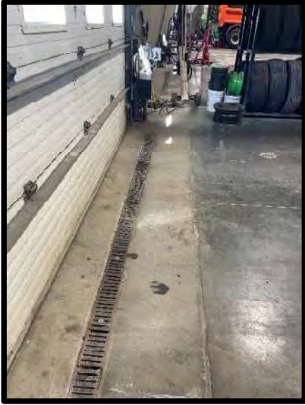
Indoor Trench Drains – 10/16/2023
