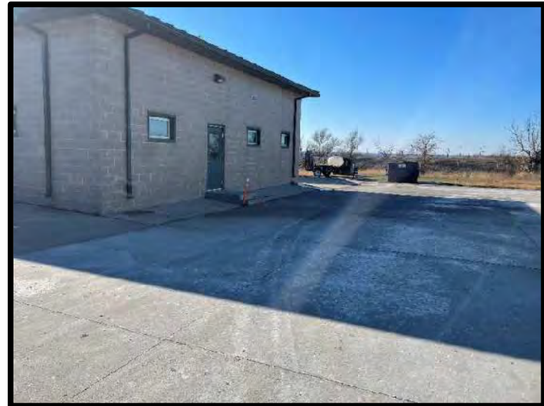
Picture 4: South Building Exterior North Face – 11/28/2023
