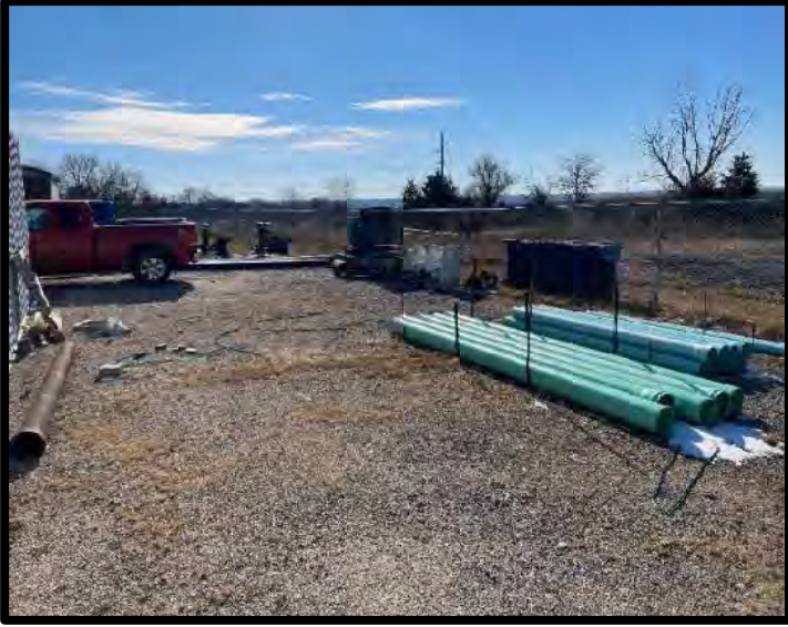
Picture 25: Outdoor Construction Material Storage – 11/28/2023
