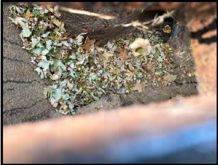
Picture 31: Interior of Inlet West of Salt Storage Building – 11/14/2023
