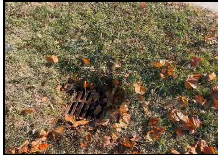
Picture 14: Area Inlet West of Main Building – 11/21/2023
