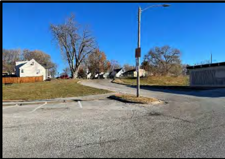
Picture 11: Parking Lot – 11/21/2023
