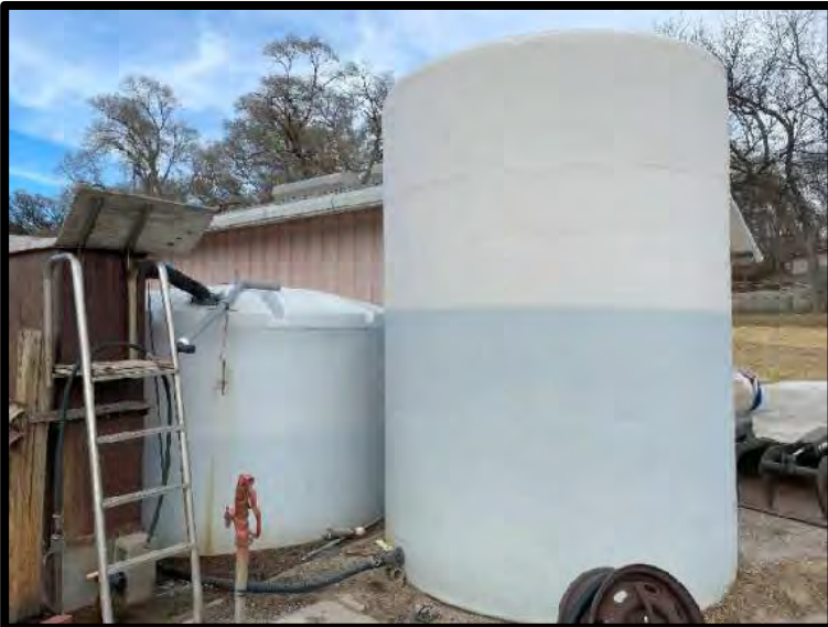
Picture 11: Liquid Storage Tanks – 11/14/2023
