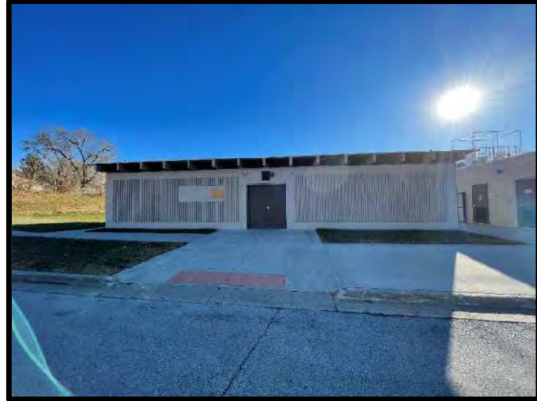
Picture 2: Main Facility Entrance – 11/21/2023
