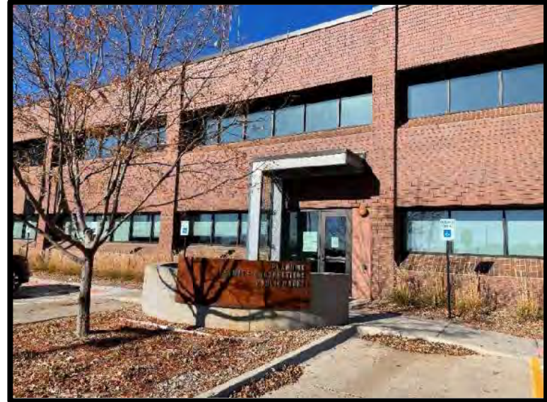
Picture 22: Public Safety Building Main Office – 11/21/2023
