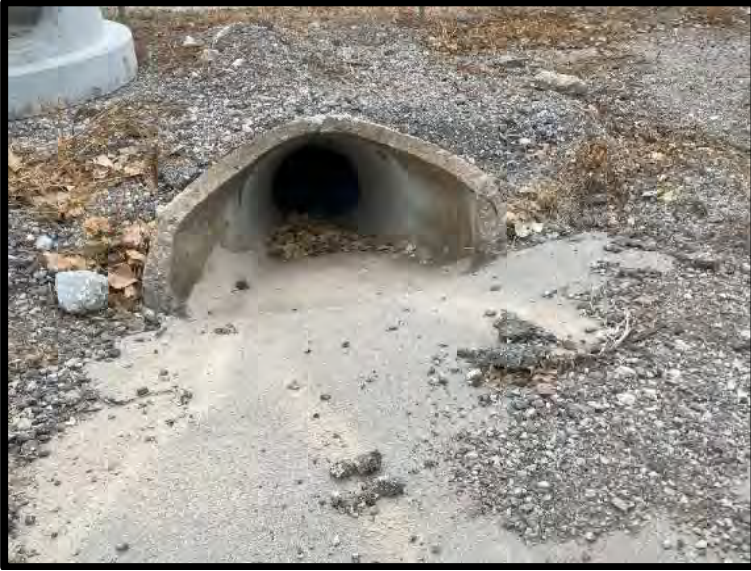
Picture 37: FES on South End of Facility – 11/16/2023
