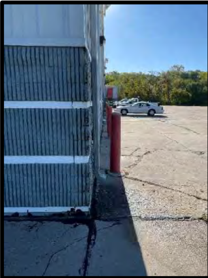
Picture 3: Downspouts South Side of Building – 10/16/2023
