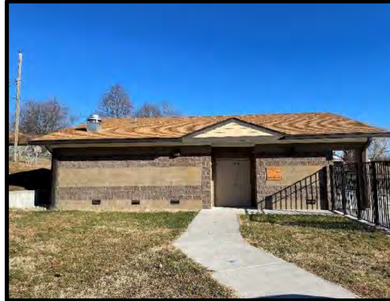
Picture 16: Entrance to Main Building – 11/21/2023
