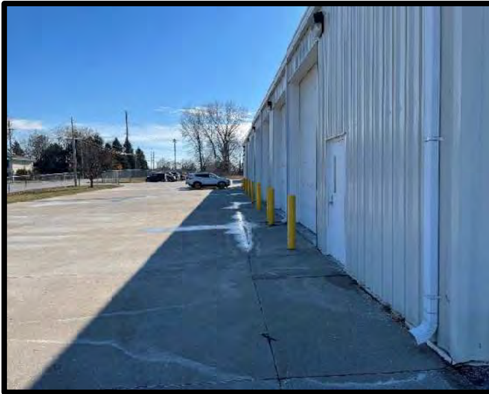
Picture 31: Downspouts on North Face of Main Office Building – 11/28/2023
