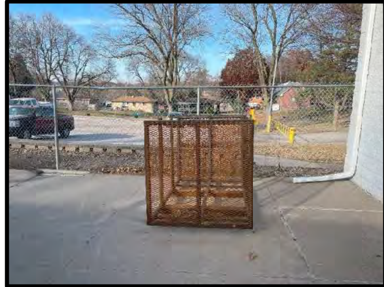
Picture 10: Downspout Drains to Impervious Surface
