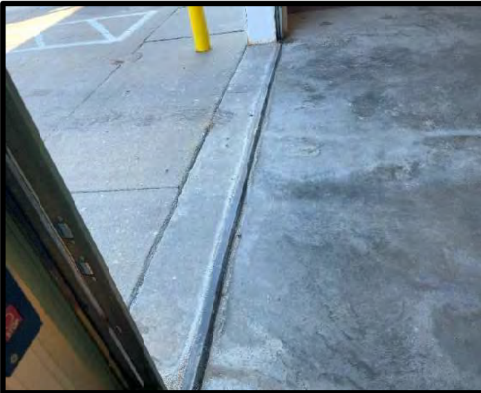
Picture 35: Berm at Garage Door Bays – Main Office Building – 11/28/2023
