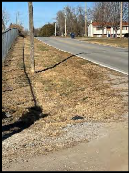
Picture 25: Drainage Swale North of Main Entrance – 11/15/2023
