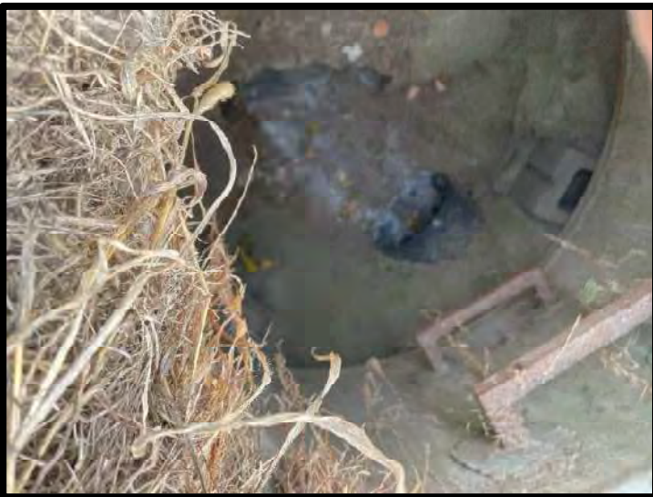
Picture 15: Interior of Area Inlet – 11/14/2023
