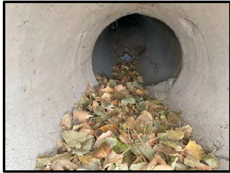
Picture 38: FES on South End of Facility – 11/16/2023
