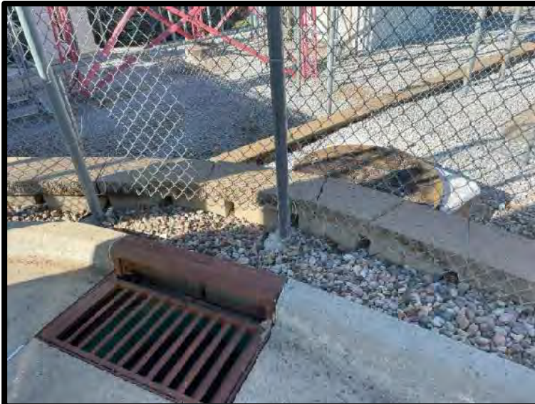
Picture 3: Area Inlet North of Facility – 11/21/2023
