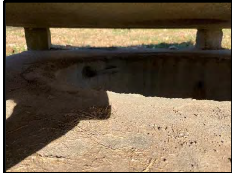
Picture 8: Area Inlet North of Facility – 11/21/2023
