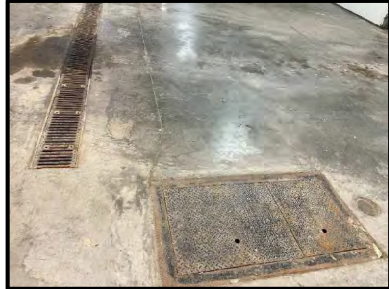
Picture 2: Trench Drain Sump Inside Main Office Garage – 11/28/2023
