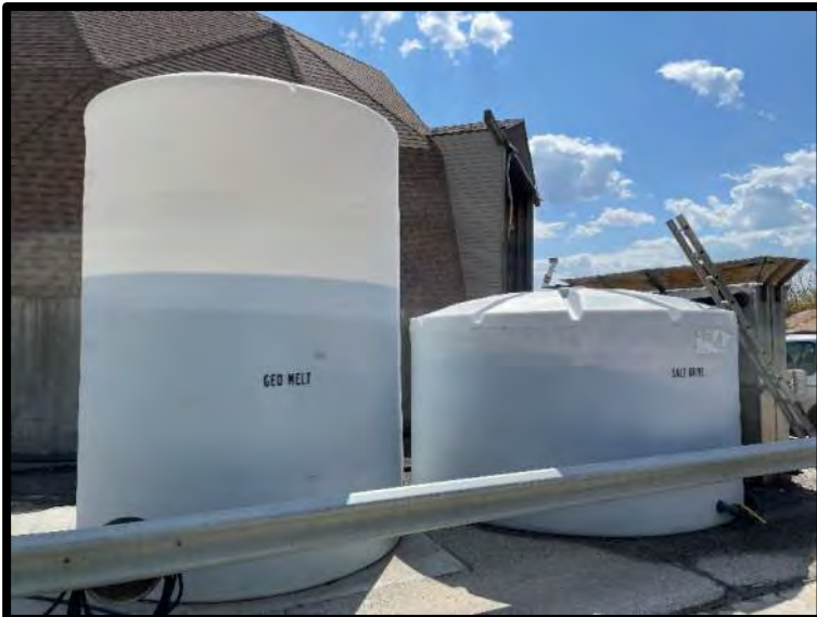
Picture 3: Liquid Deicer Tanks – 9/14/2023
