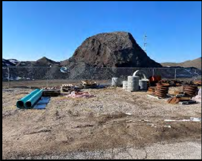
Picture 27: Outdoor Construction Material Storage – 11/28/2023
