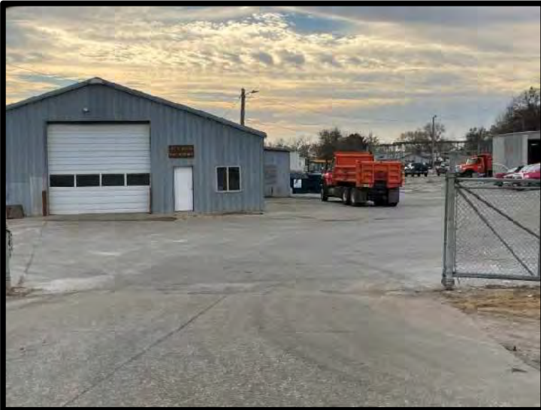
Picture 43: Main Facility Entrance – 11/16/2023
