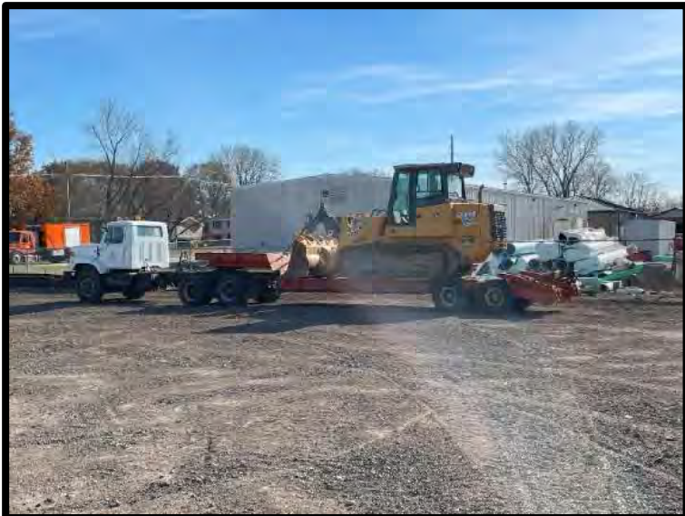
Picture 3: Vehicle and Equipment Storage – 11/15/2023
