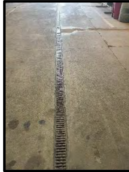
Picture 18: Main Shop Trench Drain – 11/15/2023
