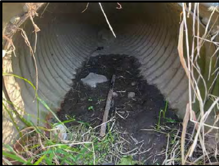
Picture 15: Culvert Outlet Southeast of Facility – 10/16/2023
