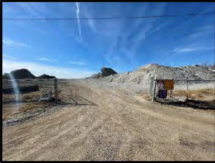
Picture 11: Site Entrance – 11/15/2023
