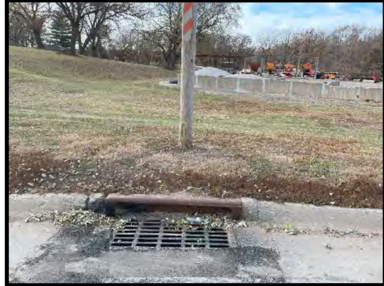
Picture 30: Inlet West of Salt Storage Building – 11/14/2023
