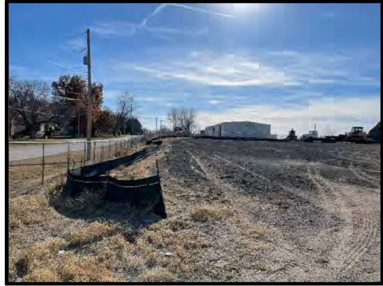
Picture 6: Silt Fence South of Entrance West of Fence – 11/15/2023
