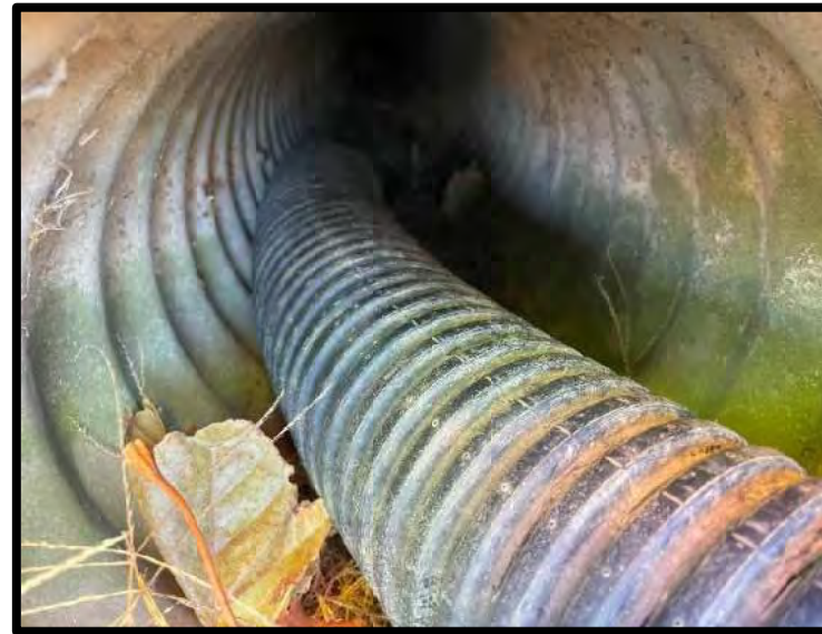
Picture 8: Culvert Inlet South of Pool – 11/21/2023
