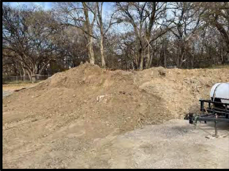
Picture 17: Soil Stockpile Storage – 11/14/2023
