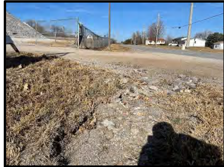
Picture 8: Culvert Outlet Under Facility Entrance – 11/15/2023
