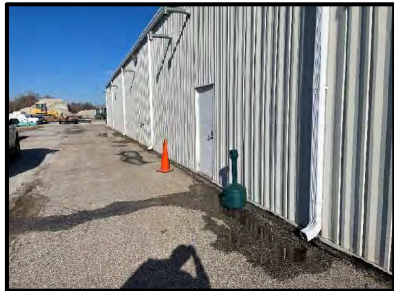
Picture 16: Concrete Parking Lot – 8/3/2022
