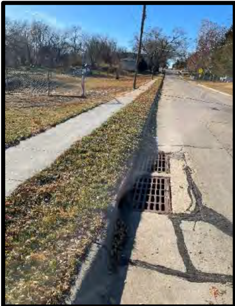
Picture 7: Area Inlet North of Facility – 11/21/2023
