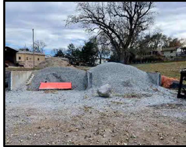
Picture 22: Outdoor Gravel Storage – 11/14/2023
