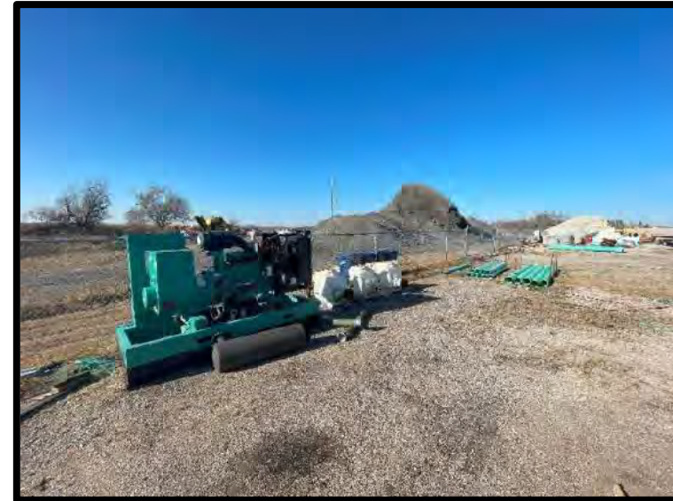
Picture 24: Outdoor Equipment Storage – 11/28/2023
