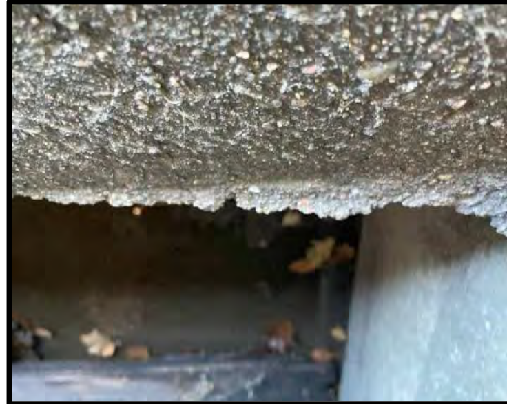
Picture 14: Inlet at Main Facility Exit – 11/21/2023
