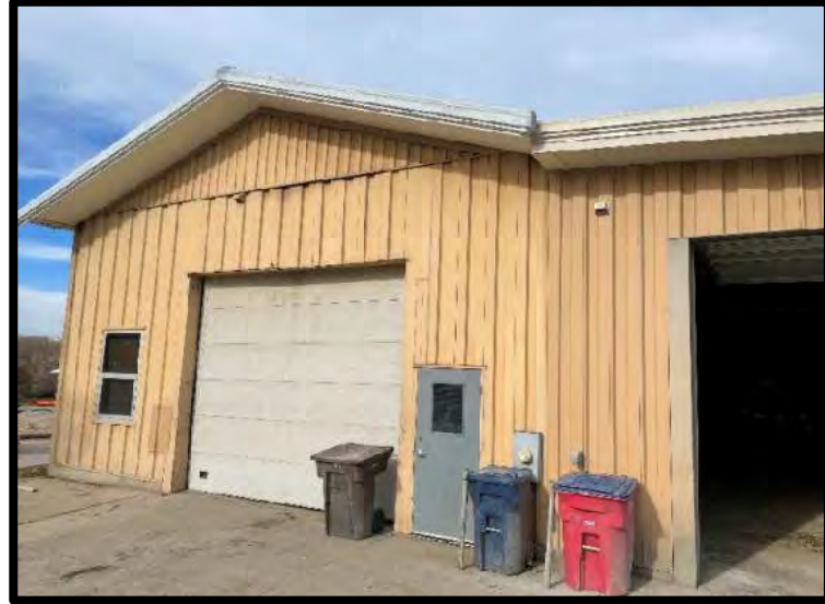
Picture 2: Exterior of Main Office Building – 11/14/2023
