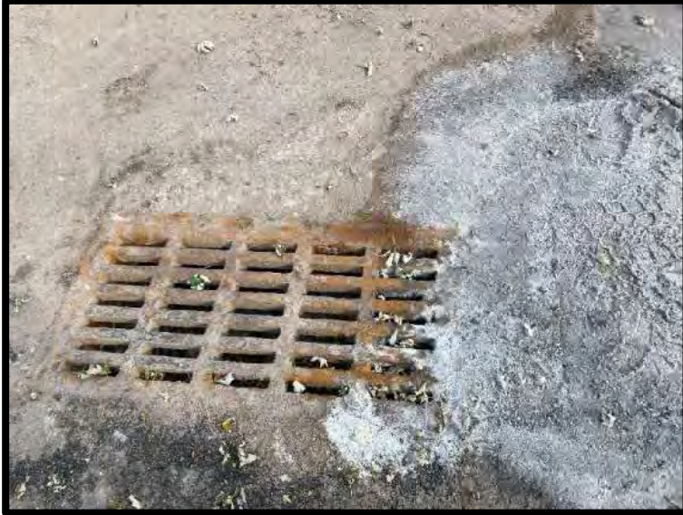
Picture 29: Winter Mix Entering Inlet at Salt Storage Building – 11/14/2023
