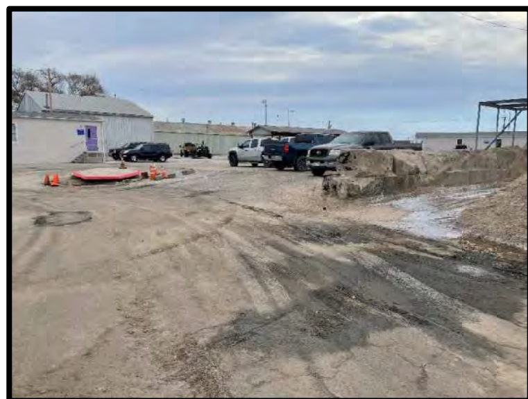
Picture 28: Stains Leading to Area Inlet – 11/16/2023
