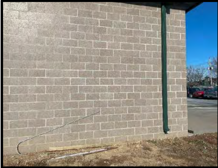
Picture 7: South Building Exterior South Face – 11/28/2023
