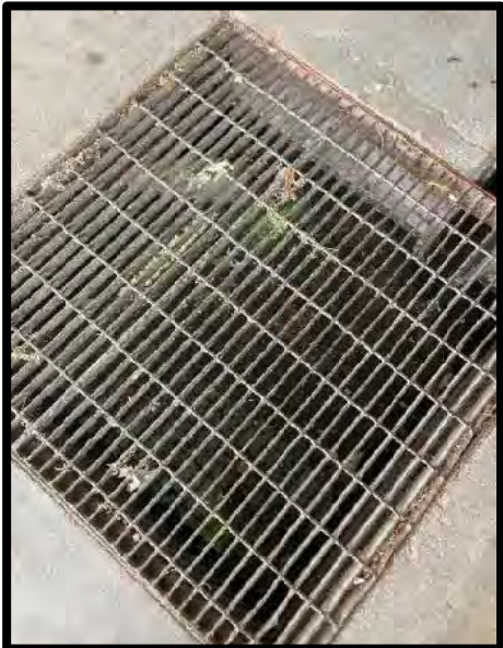
Picture 19: Main Shop Drain Pit – 11/15/2023
