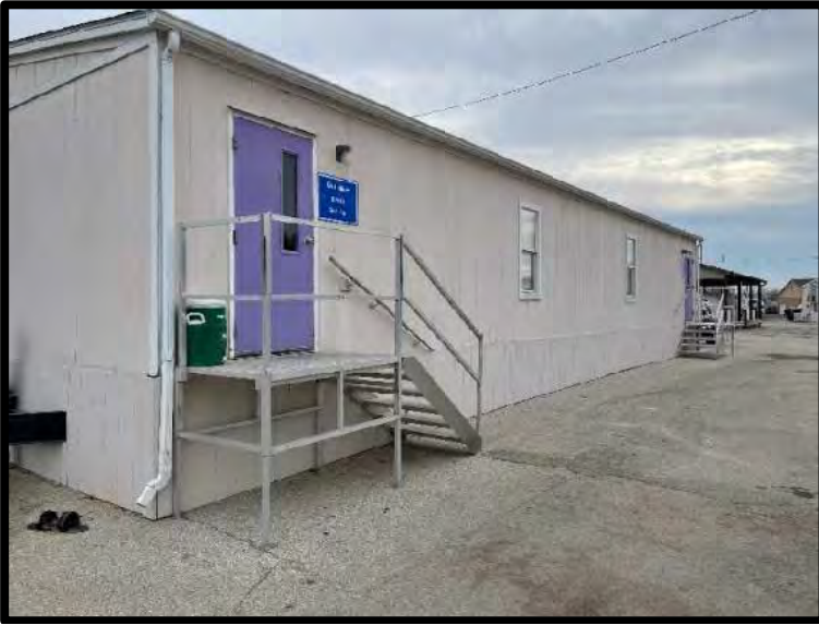
Picture 9: Sign Shop and Breakroom Building – 11/16/2023
