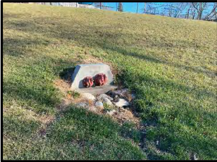
Picture 5: Pool Drainage North Outlet – 11/21/2023
