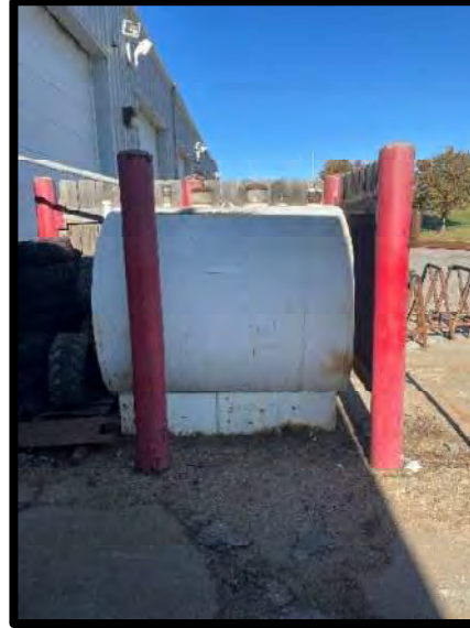
Picture 6: Outdoor Used Oil Storage Tank – 10/16/2023
