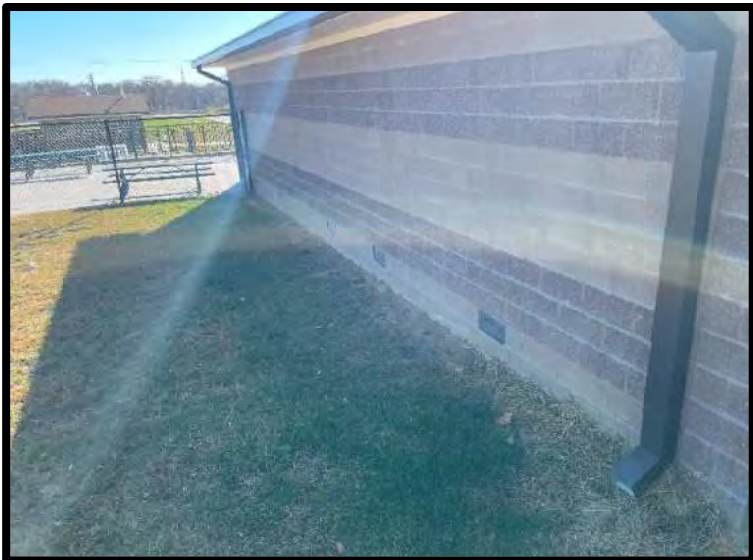
Picture 3: Downspouts on East Side Main Building – 11/21/2023
