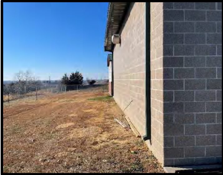
Picture 5: South Building Exterior South Face – 11/28/2023
