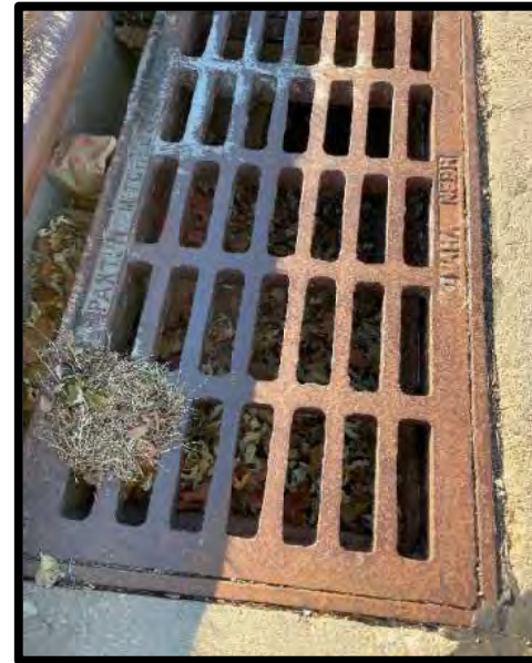
Picture 8: Area Inlet North of Facility – 11/21/2023
