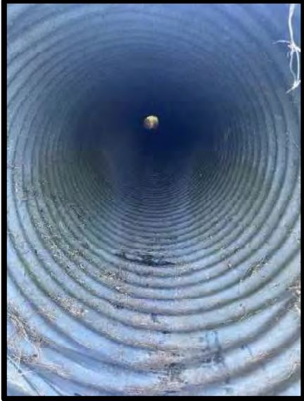
Picture 13: Culvert Interior Southeast of Facility – 10/16/2023
