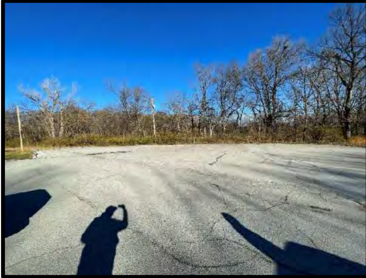
Picture 1: Parking Lot – 11/21/2023
