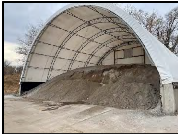
Picture 20: Salt Stockpile – 11/16/2023
