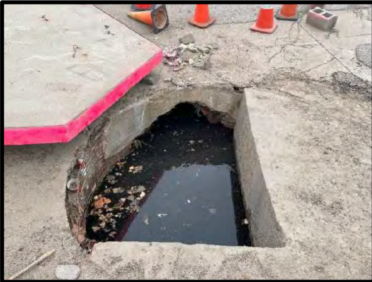
Picture 7: Area Inlet at Center of Facility – 11/16/2023
