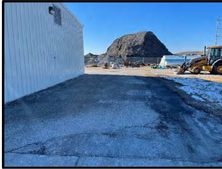
Picture 30: Pavement North of Main Office Building – 11/28/2023
