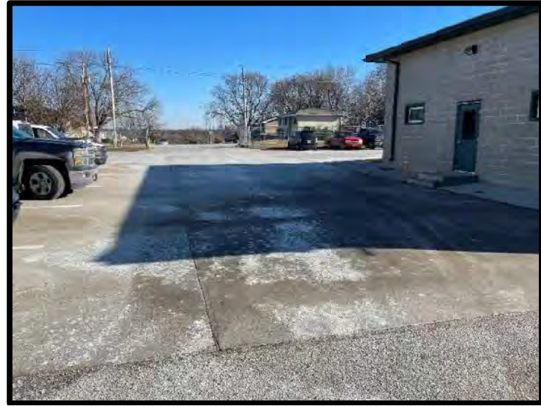
Picture 18: Paved Area North of Main Building – 11/28/2023
