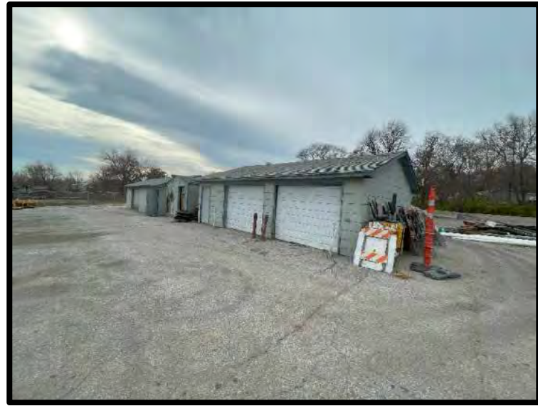
Picture 42: Storage Sheds Southwest Corner of Facility – 11/16/2023
