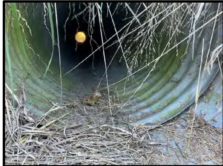
Picture 16: Culvert Interior Southwest of Facility – 10/16/2023
