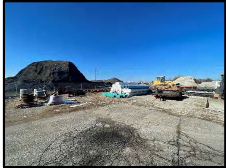
Picture 28: Outdoor Construction Material Storage – 11/28/2023
