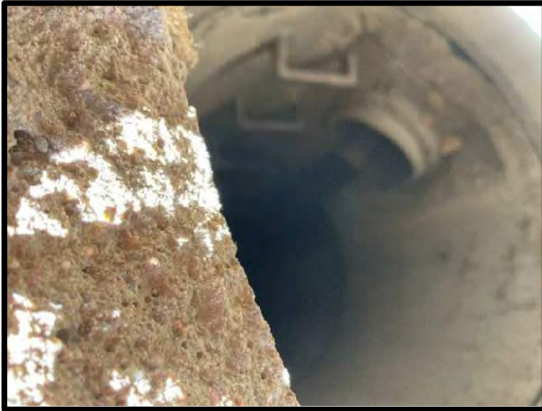
Picture 9: Area Inlet North of Facility – 11/21/2023
