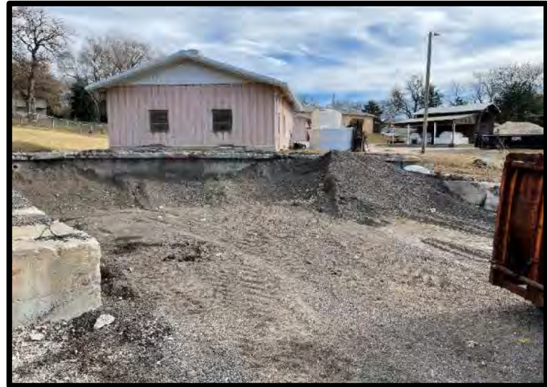
Picture 16: Asphalt Millings Storage – 11/14/2023
