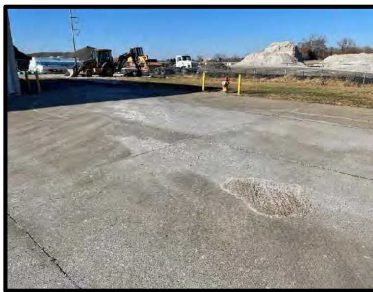
Picture 32: Concrete Parking Lot – 8/3/2022
