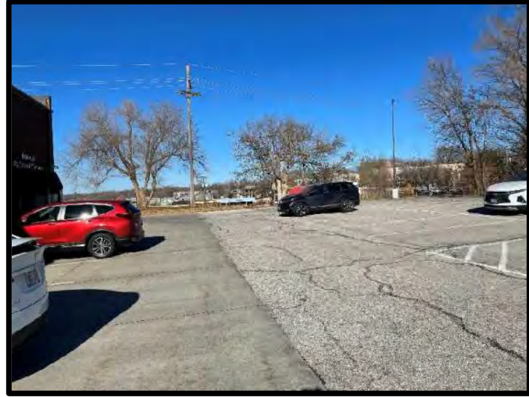
Picture 6: General Parking Lot East of Administrative Office – 11/21/2023
