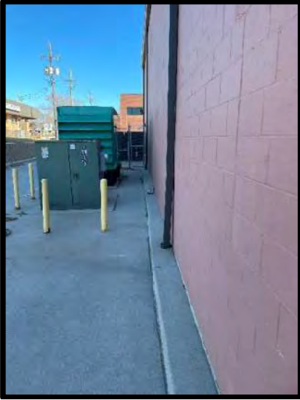
Picture 5: Downspouts Diverted North of Facility – 11/21/2023
