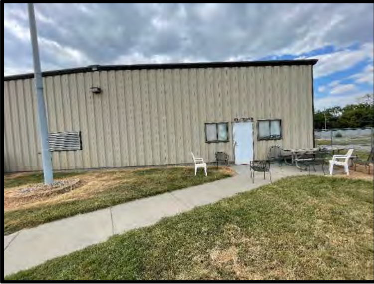
Picture 13: Front of Facility/Main Office – 9/14/2023
