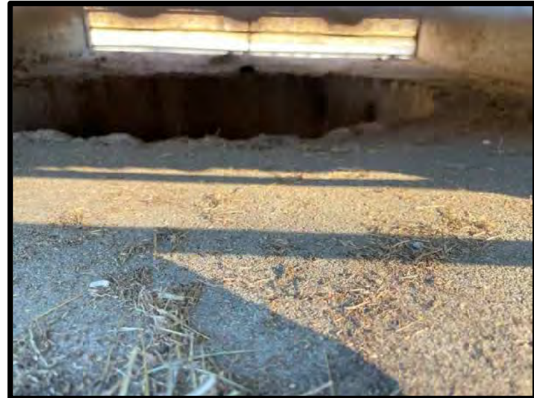
Picture 4: Area Inlet Southeast of Facility – 11/21/2023
