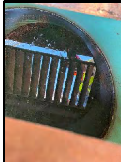
Picture 4: Interior of Area Inlet North of Facility – 11/21/2023
