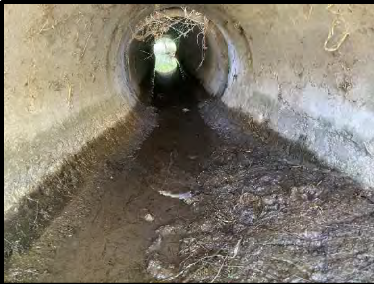
Picture 11: Culvert Interior Northeast of Facility – 10/16/2023
