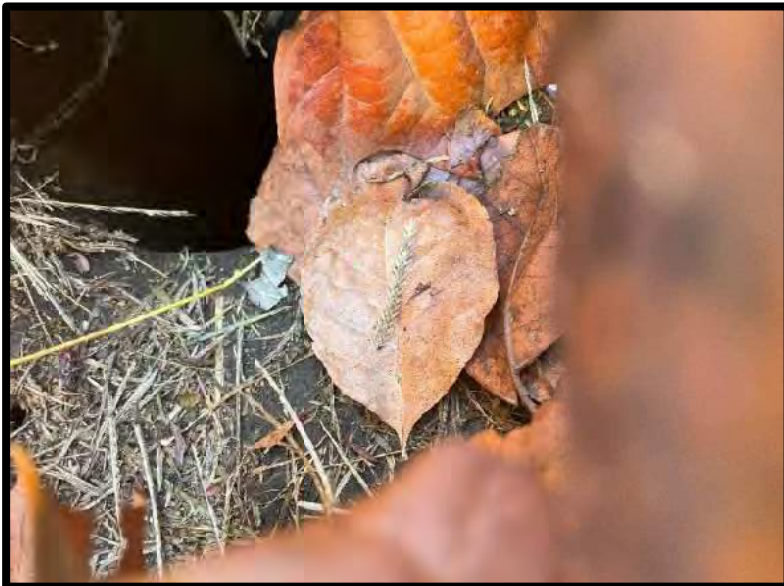
Picture 15: Area Inlet West of Main Building – 11/21/2023
