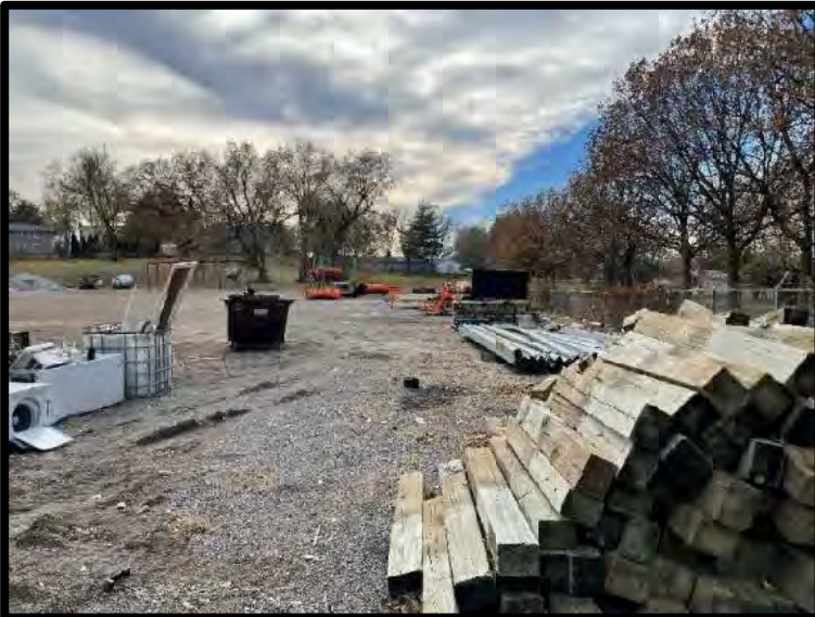
Picture 19: Construction Material Storage – 11/14/2023
