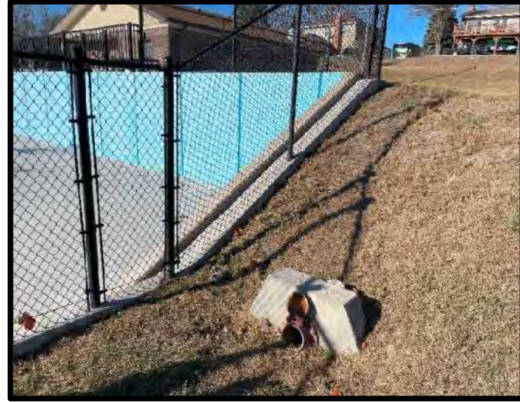
Picture 6: Floor Drain Outlet East of Pool – 11/21/2023
