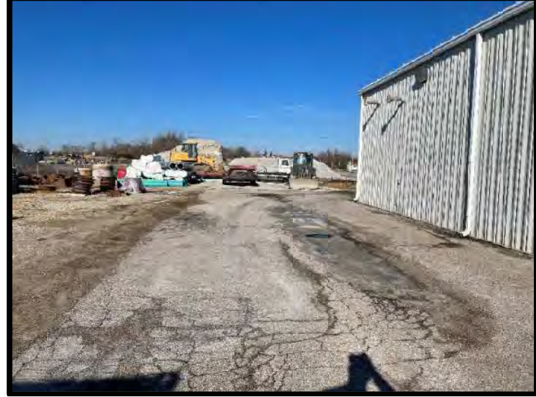
Picture 26: Paved Area West of Main Office Building – 11/28/2023
