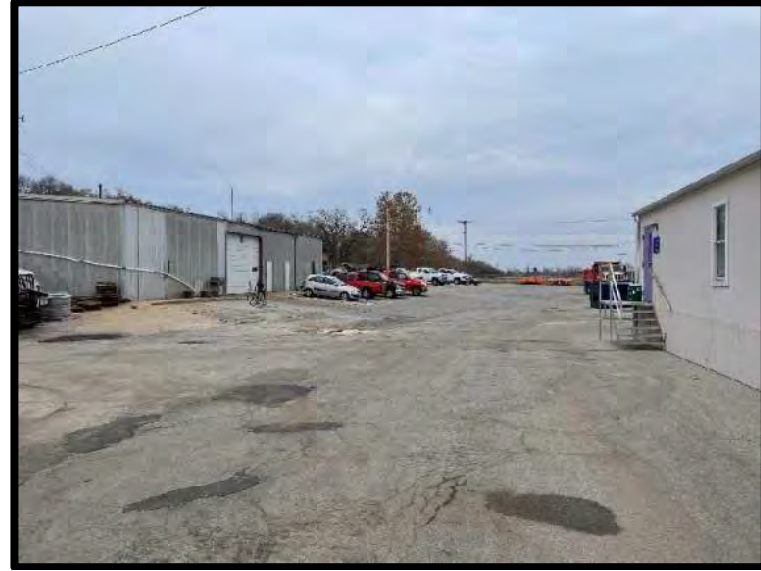
Picture 6: Paved Area West of Sign Shop and Breakroom Building – 11/16/2023
