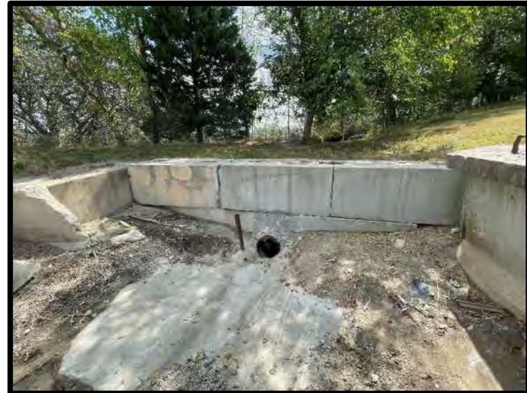
Picture 8: Stormwater Drainage Culvert – 9/14/2023
