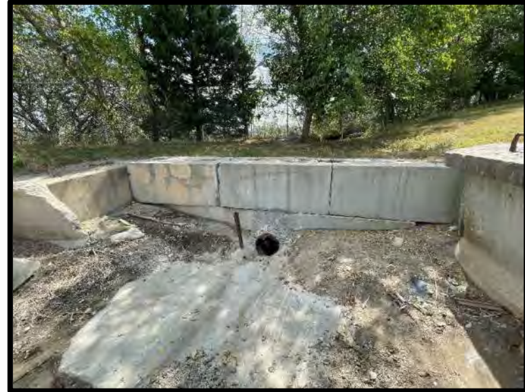
Picture 8: Stormwater Drainage Culvert – 9/14/2023
