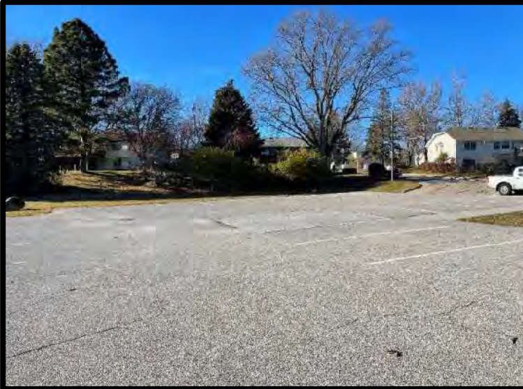
Picture 11: Parking Lot – 11/21/2023
