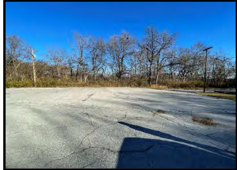
Picture 2: Parking Lot – 11/21/2023
