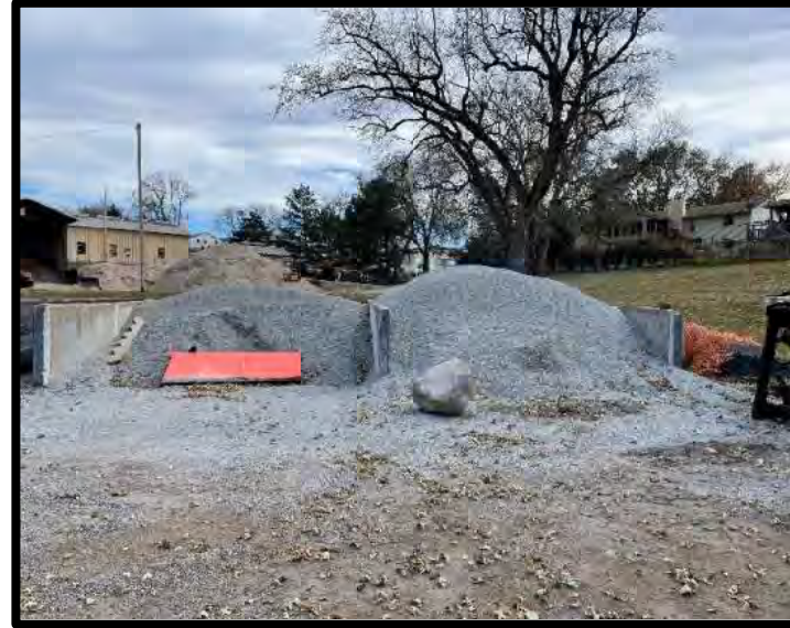
Picture 22: Outdoor Gravel Storage – 11/14/2023
