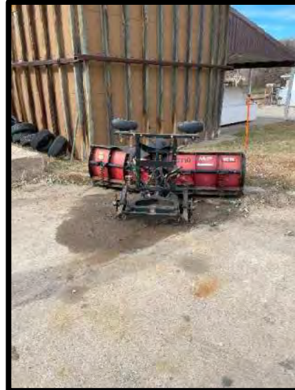
Picture 4: Stains Near Plow Storage, SW of Salt Storage Building – 11/14/2023
