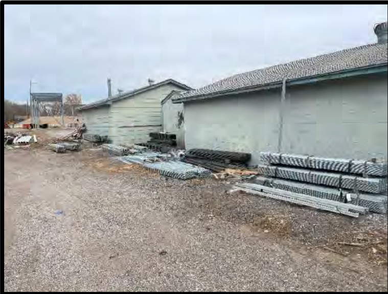
Picture 39: Material Storage West of Storage Sheds – 11/16/2023
