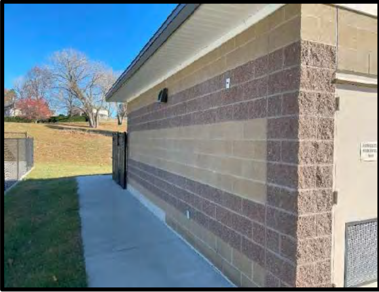
Picture 9: North Side of Pump Building – 11/21/2023
