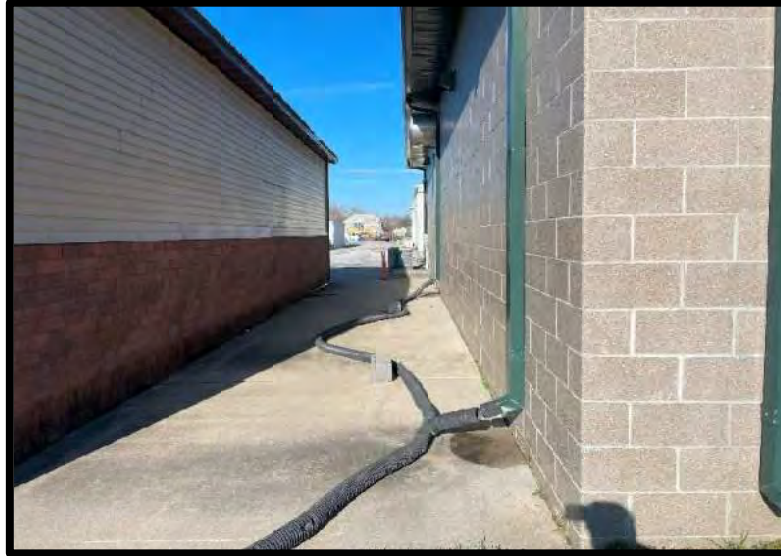
Picture 8: South Building Exterior West Face – 11/28/2023
