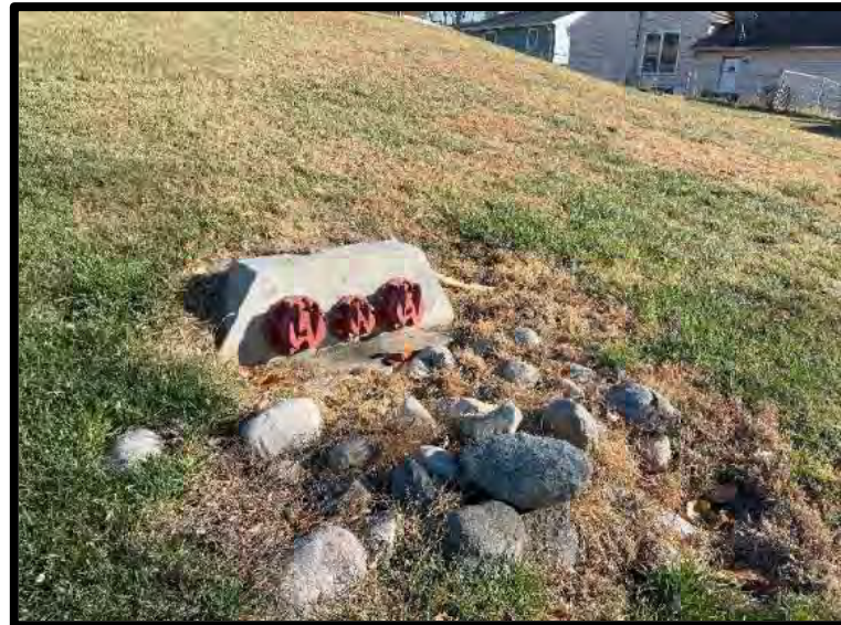
Picture 4: Pool Drainage South Outlet – 11/21/2023
