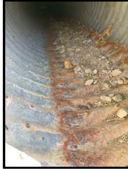
Picture 10: Interior of Culvert Crossing Cedar Island Road – 11/15/2023
