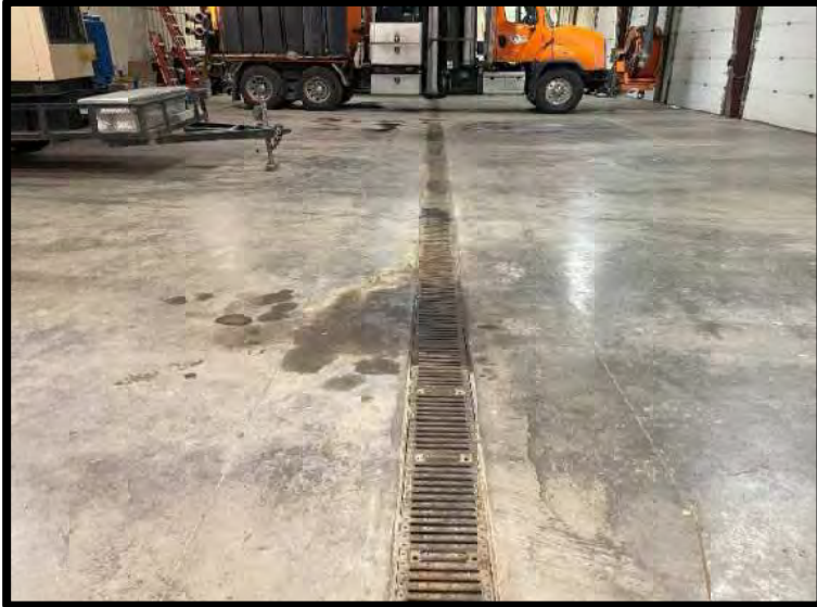
Picture 1: Trench Drain Inside Main Office Garage – 11/28/2023
