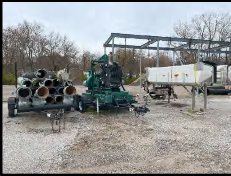
Picture 41: Outdoor Equipment Storage – 11/16/2023
