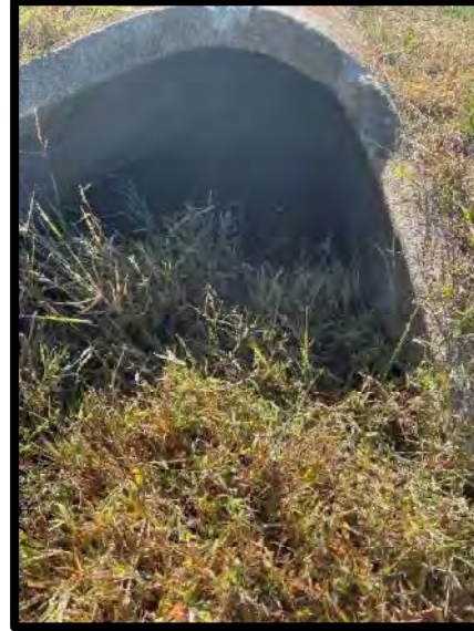
Picture 10: Culvert Inlet Northeast of Facility – 10/16/2023
