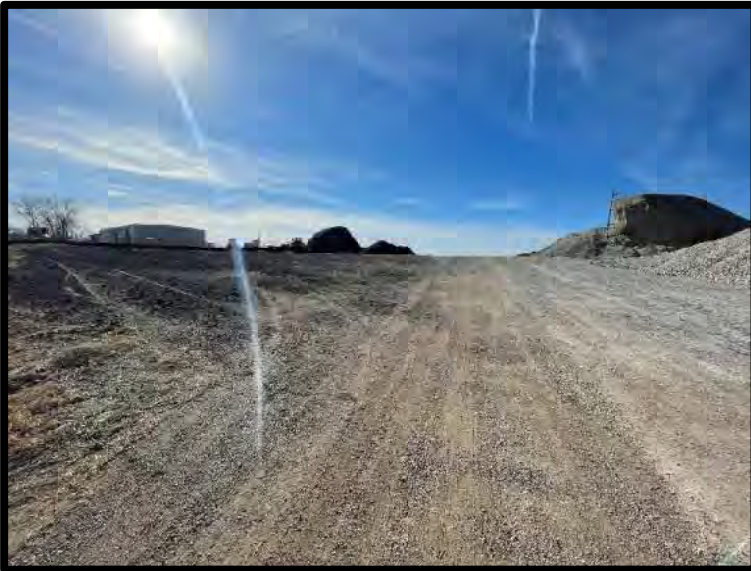
Picture 7: Main Entrance to Facility
