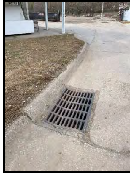
Picture 6: Inlet West of Sand/Gravel Storage – 11/14/2023
