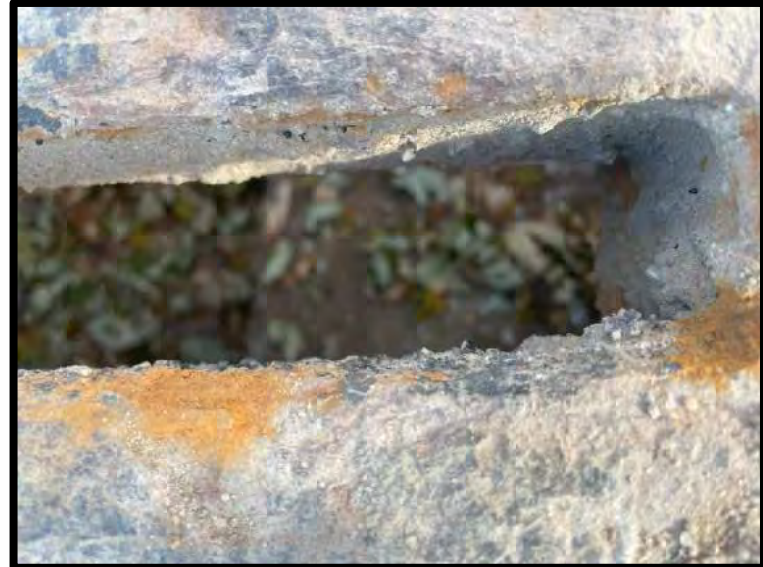
Picture 28: Interior of Inlet near Salt Storage – 11/14/2023
