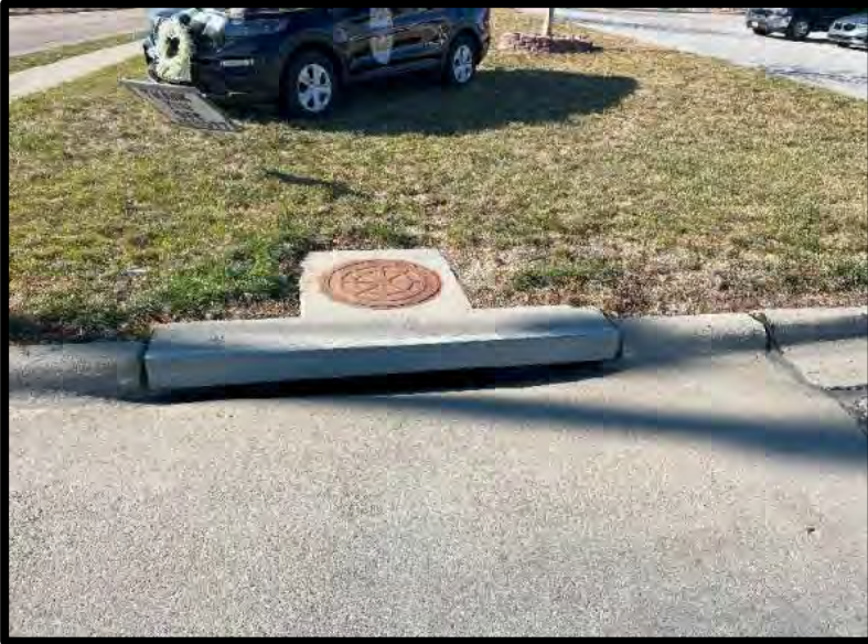
Picture 13: Inlet at Main Facility Exit – 11/21/2023
