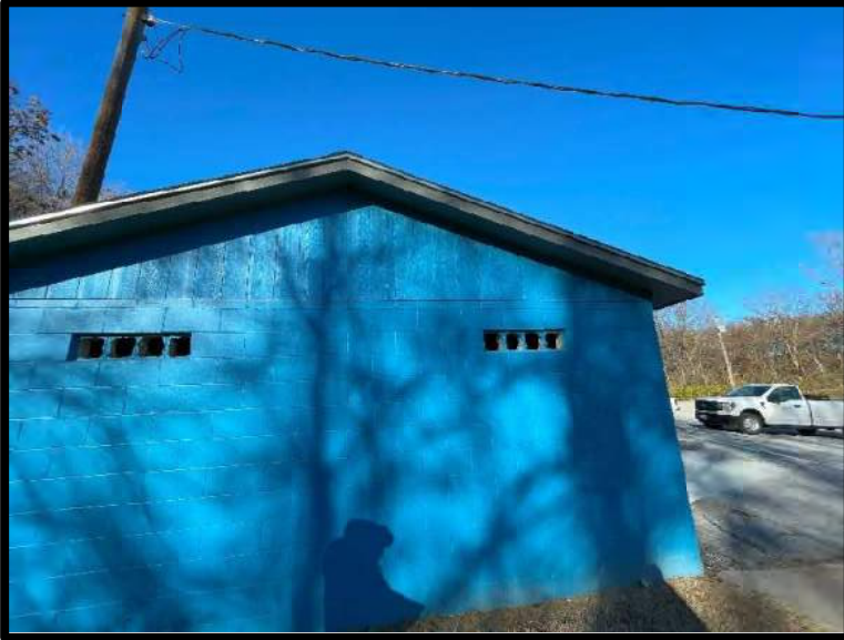
Picture 5: South Wall of Pump Building – 11/21/2023
