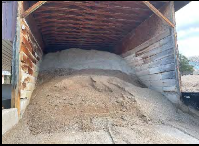
Picture 25: Salt Storage Building – 11/14/2023
