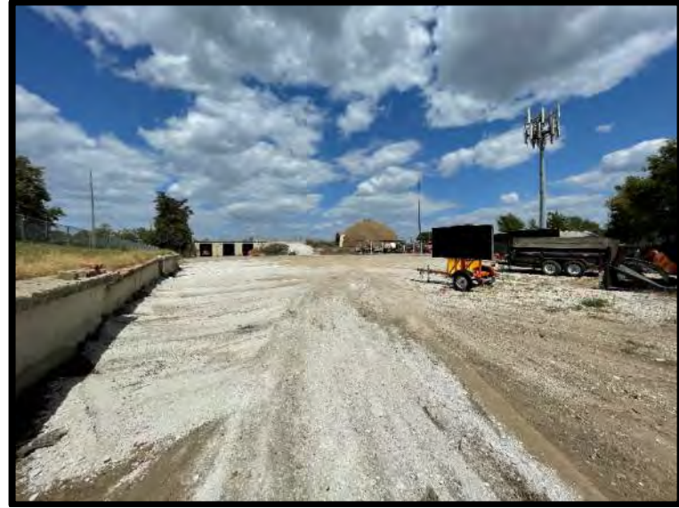
Picture 10: Drainage Area to Culvert Pipe – 9/14/2023
