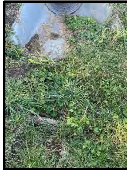
Picture 14: Culvert Inlet Southeast of Facility – 10/16/2023
