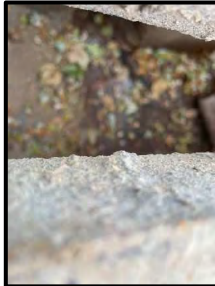
Picture 12: Interior of Vehicle Washout Inlet – 11/14/2023
