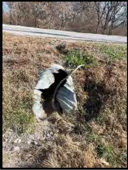
Picture 9: Culvert Inlet Crossing Cedar Island Road – 11/15/2023
