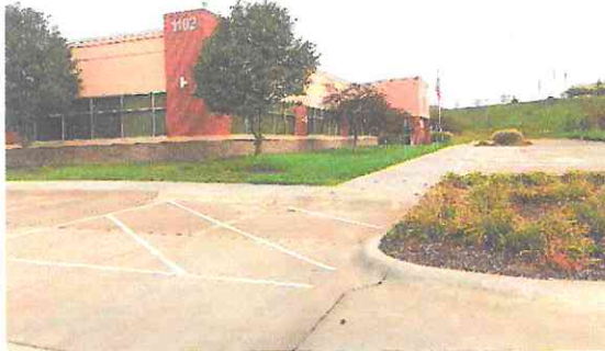
Photo #1: East side of building/main entrance, looking north.
