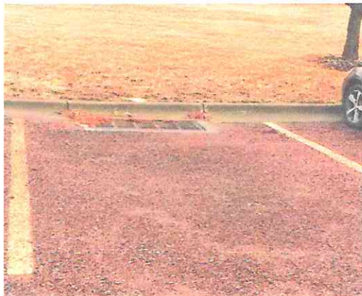
Photo #5 Storm Drain Inlet - Southwest Parking Lot
