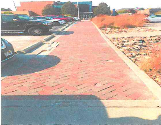
Photo #9: Green infrastructure system with impervious pavers and water-wise landscaping in front of treasurer's office.
