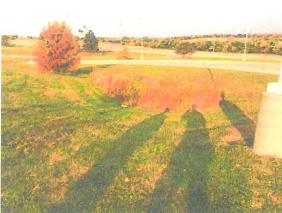
Photo #21: Small Bioretention Cell #1 taking Drainage from North Parking Area.
