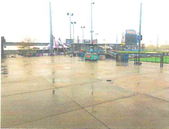
Photo #3: Left Field Terrace area, looking north.
