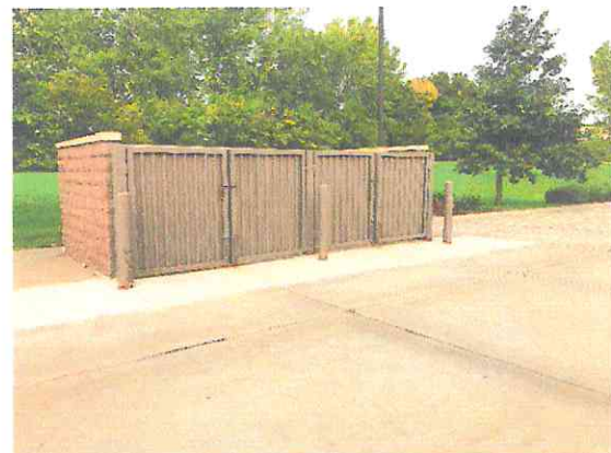
Photo #12: Solid waste dumpster enclosure, west side of building.
