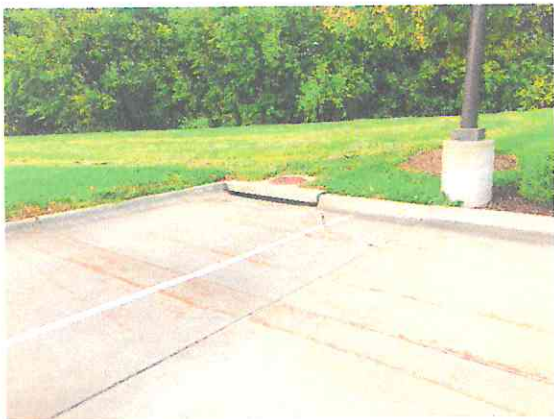
Photo #15: Storm drain inlet (south), west parking area.
