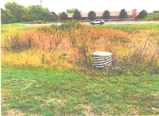
Photo #7: Detention basin on south side of property, looking north.
