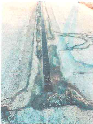
Photo #17: Ground Drain near Gold Coast Storage Facility-East Driveway
