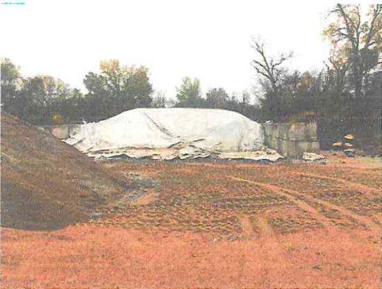
Photo #3: Road salt stockpile covered in a dedicated bay.
