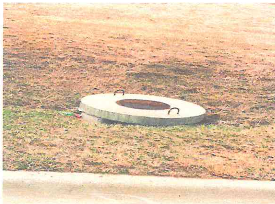
Photo Photo #17: Site Castletop Drain17
