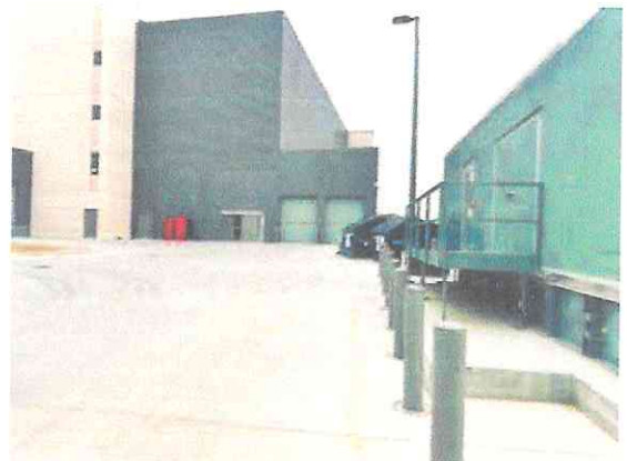
Photo #18: Parking Lot Area, North of jail where Generator and waste containers and Sally Port are located
