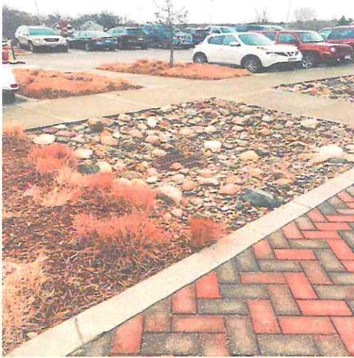
Photo- #19: Administration Parking Lot East Drainage System
