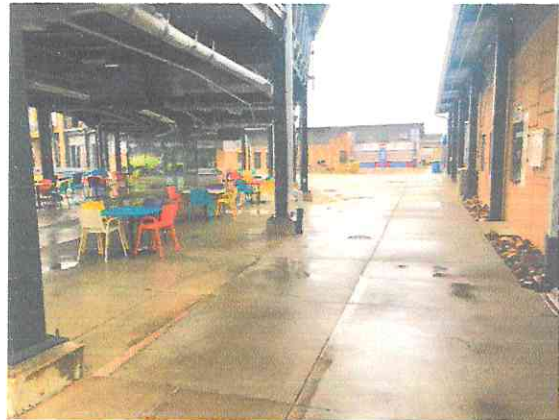
Photo #2: Main concourse, 3 rd base side, looking south.
