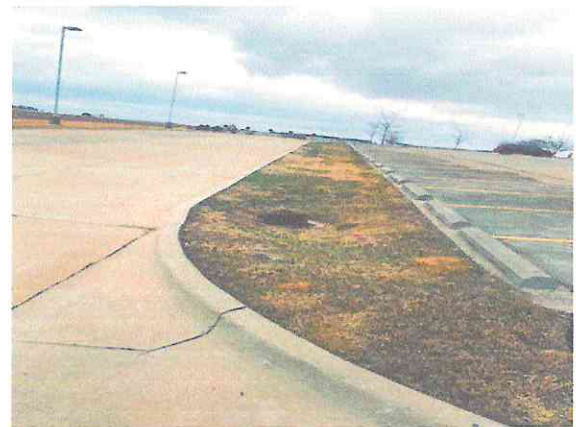
Photo #16: Parking Lot Drainage
