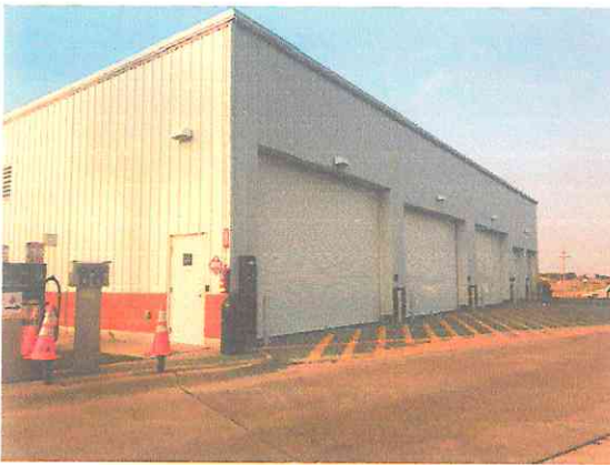
Photo #9: Cold Storage Building, South Side of Property
