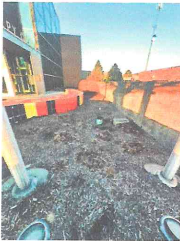
Photo #15: Ground Drain near North Side of East Annex Building
