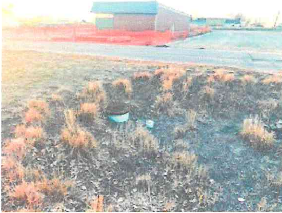
Photo #7: Bioretention cell located on the south side of the east parking lot.
