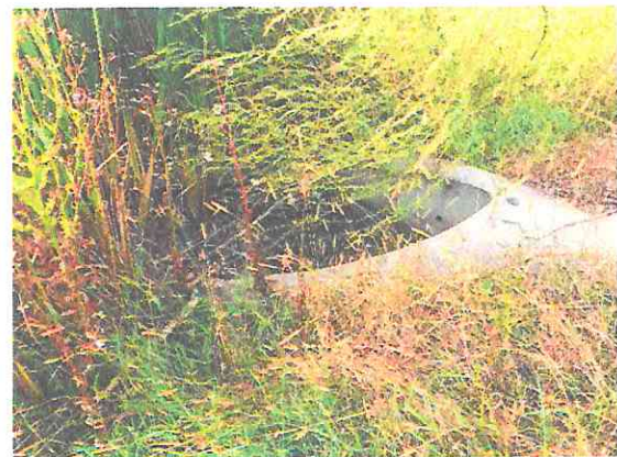
Photo #6: Detention basin inlet
