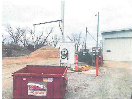
Photo #2: 500 gallon AST fueling area, and two-bay garage & cold storage building.
