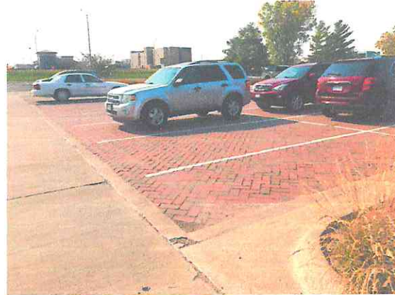
Photo #8: Pervious pavers in an area of the southeast parking lot
