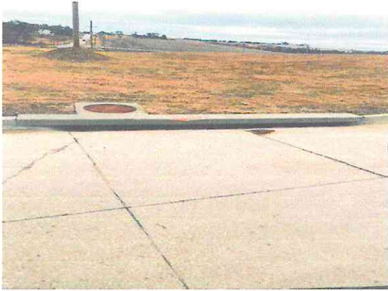
Photo #13: Storm Water Drainage Inlet
