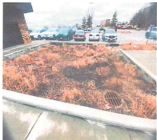
Photo #24: Greenspace Drainage - East Annex - Additional Photo
