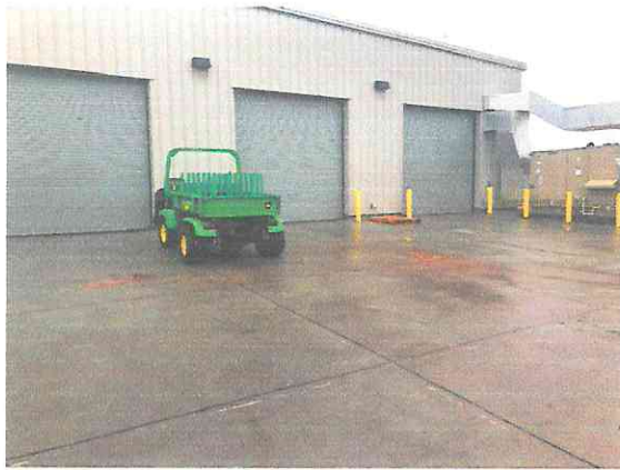
Photo #7: Maintenance shop & cold storage, beyond left field area.
