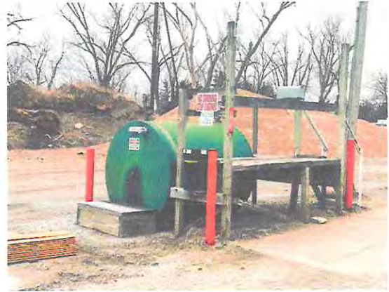
Photo #8: Fueling Station
