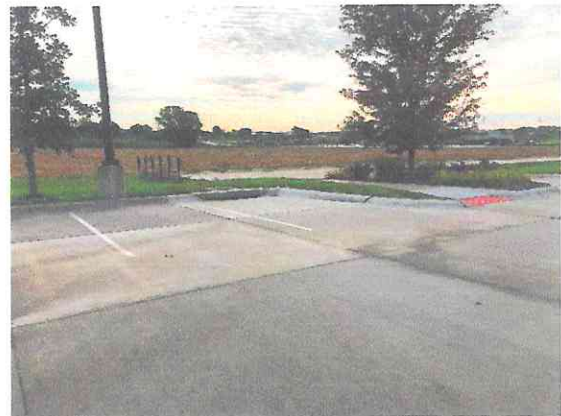
Photo #4: Storm drain inlet (south), east parking area, looking southeast.
