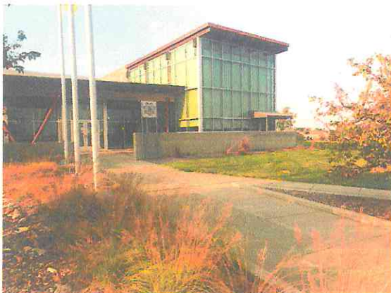
Photo #19: Main entrance to Sheriff Department Building
