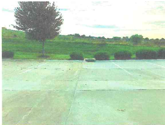
Photo #3: Storm drain inlet (north), east parking area, looking east.
