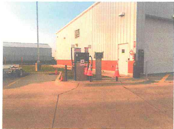
Photo #10: Fueling Area with Underground Storage Tank, Cold Storage Building
