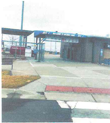
Photo #13: West Entrance to Facility
