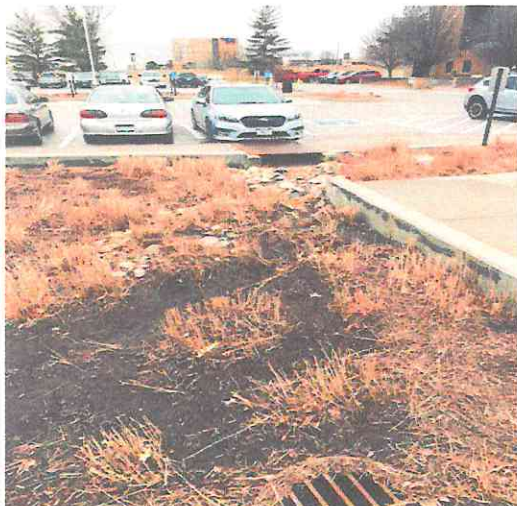
Photo #23: Greenspace Drainage - East Annex
