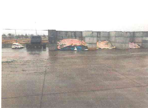
Photo #6: Covered stockpiles of field materials covered at all times when not in use.
