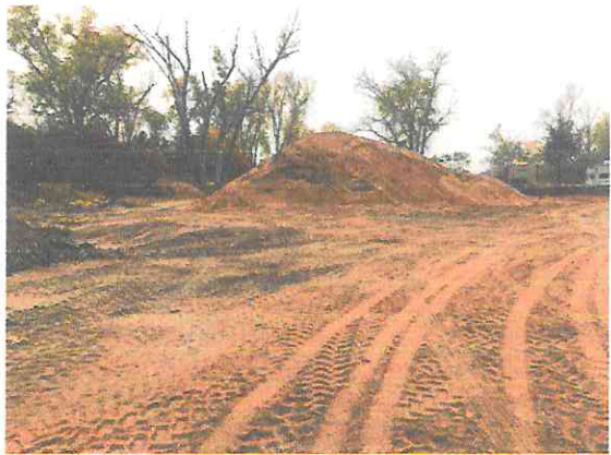
Photo #6: Sand stockpile on western edge of the facility.
