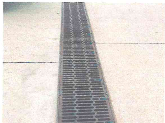
Photo #12: Outdoor Floor Drain at Center of Main Parking Area
