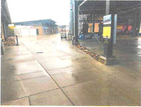
Photo #1: Main concourse, 3 rd base side, looking north.
