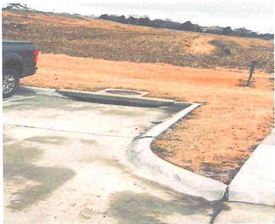
Photo #16: Storm drain inlet, east parking area.
