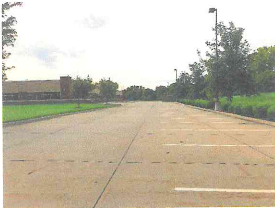
Photo #13: West parking area, looking south.
