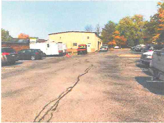
Photo #1: Parking lot leading to garage, looking north.
