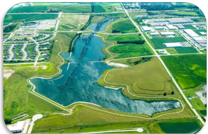
Program Project (DS-15A) after completion
