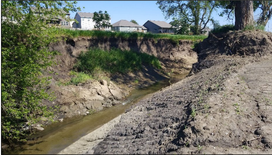
Photograph D2-1. Existing Conditions at S-5
