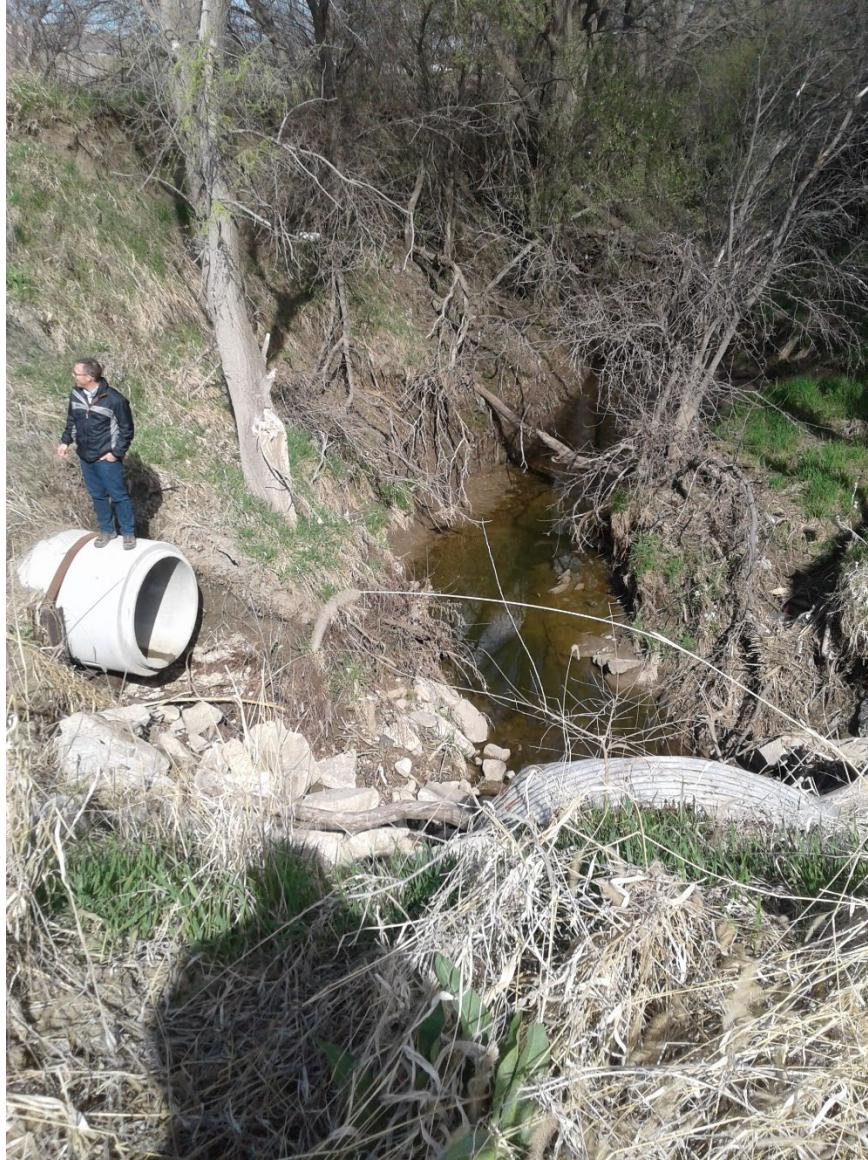
Figure 10. Upstream inlet to Beetle Creek culvert
