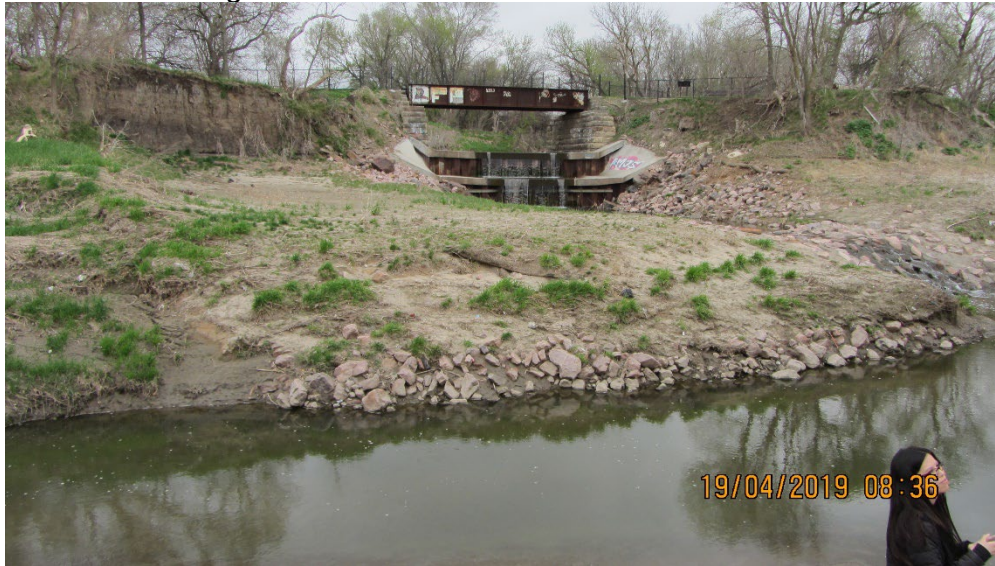
Figure 1. Hell Creek outlet structure
