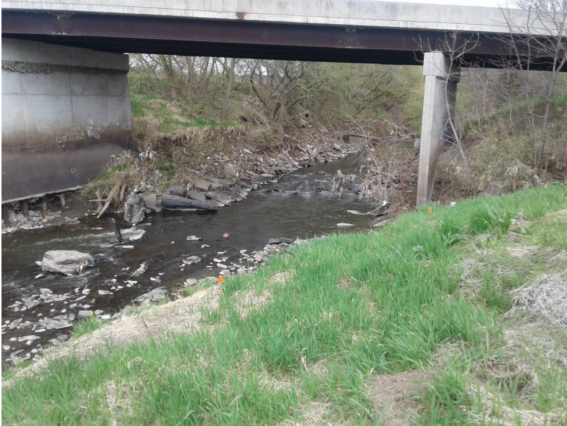
Figure 14. 132 nd St. Bridge over West Papillion Creek.
