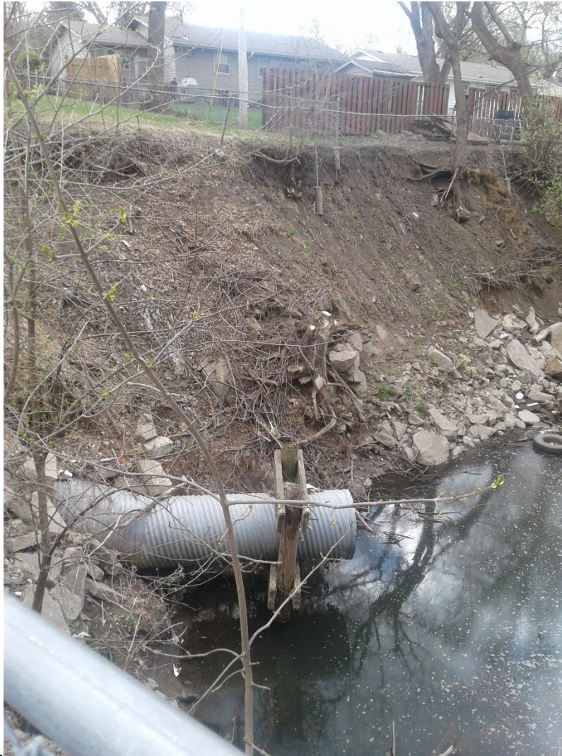
Figure 16. Bank erosion along Cole Creek results in fences and trees falling into the creek.
