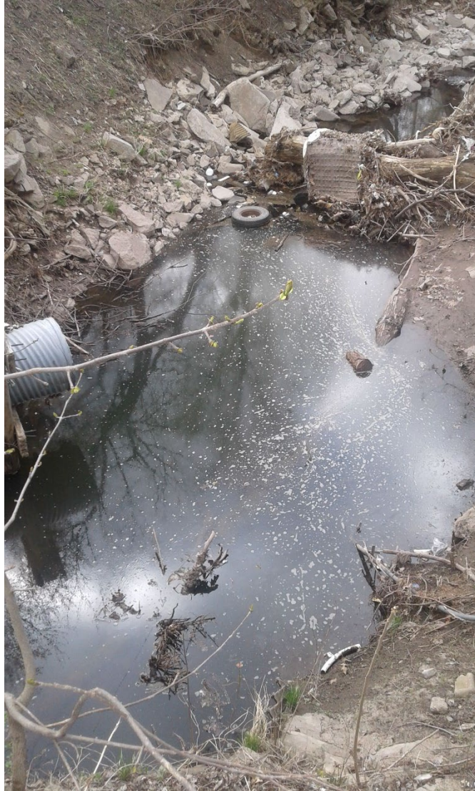
Figure 18. Cole Creek channel below Hillside Drive culvert.
