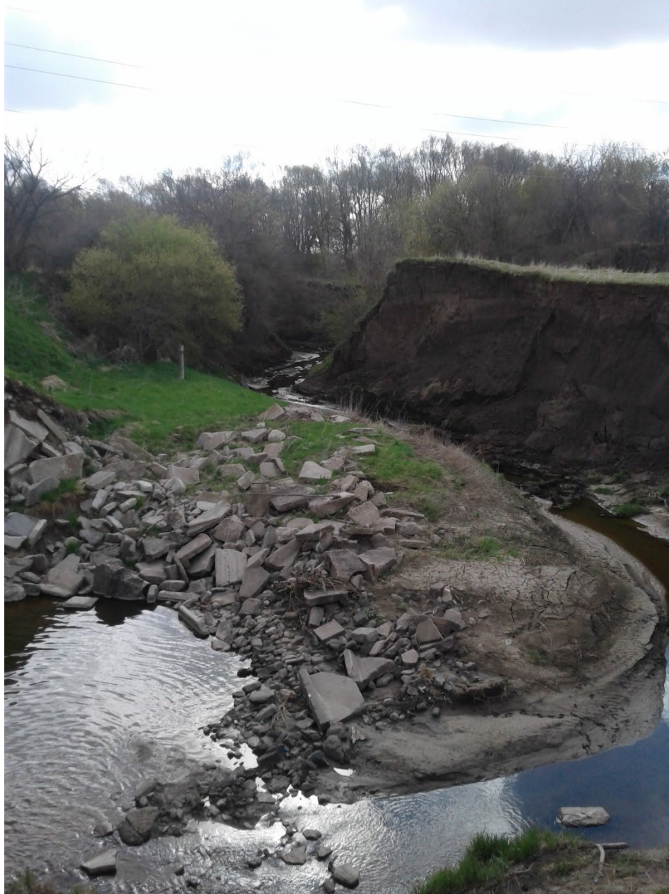
Figure 11. Outlet of Beetle Creek culvert
