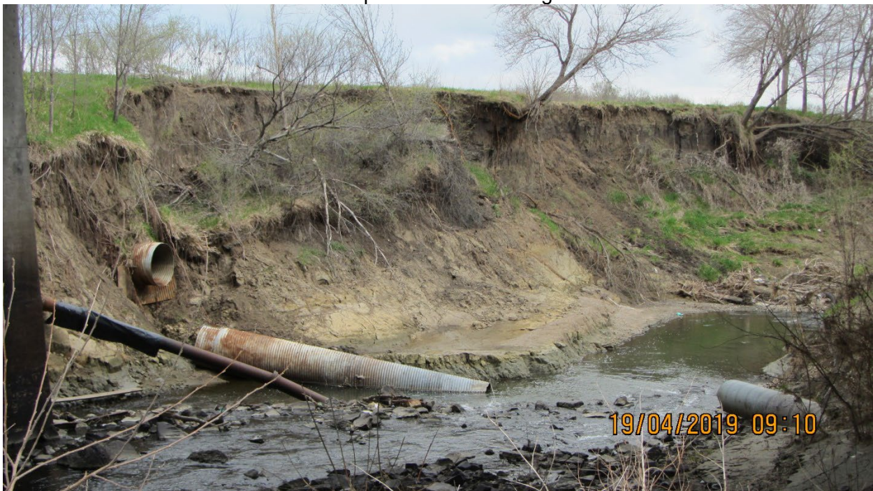
Figure 4. South Papillion Creek channel at the downstream side of Giles Road Bridge (looking downstream)
