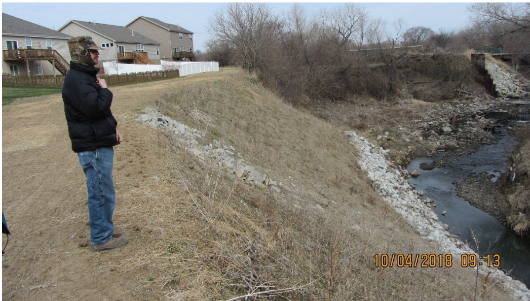
Figure 6. Newly constructed right bank slope and toe to protect sewer line (looking upstream)
