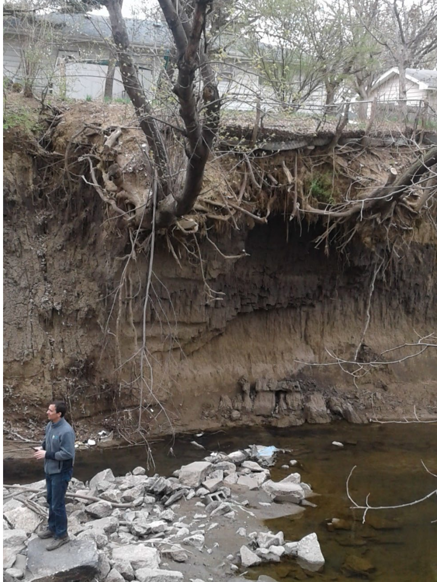
Figure 17. Cole Creek left bank failure.
