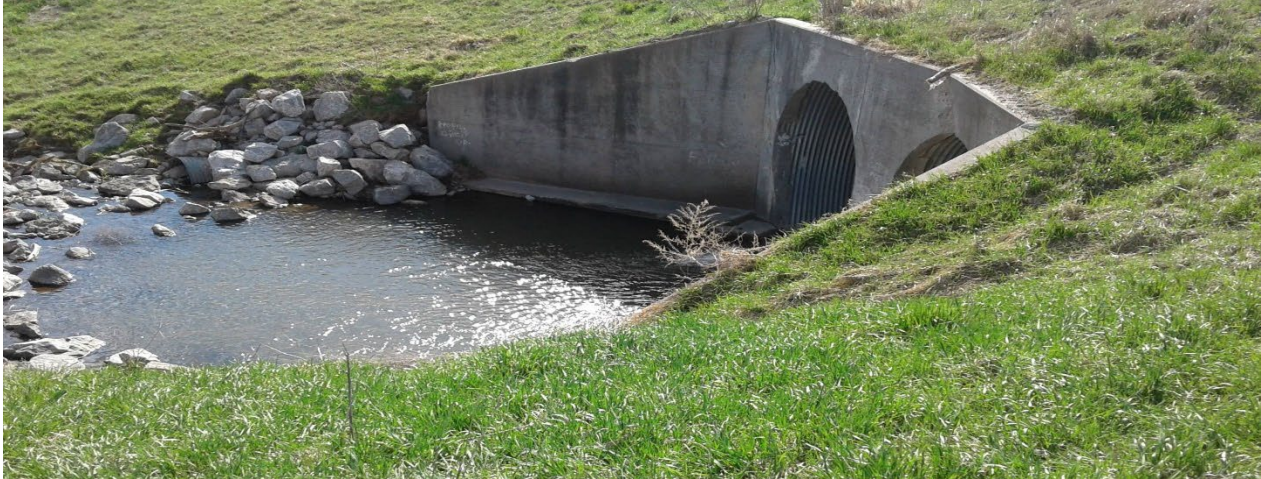
Figure 12. Culvert structure at Giles Rd. Upstream limit of site.
