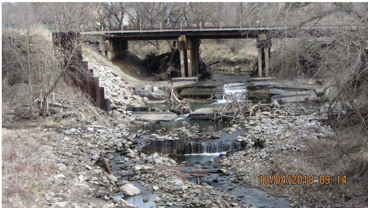
Figure 7. Railroad Bridge just east of 156 th St. (looking upstream)
