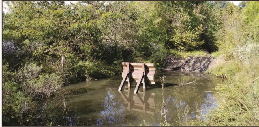
Figure 6. Campbell Creek grade control structure #1.
