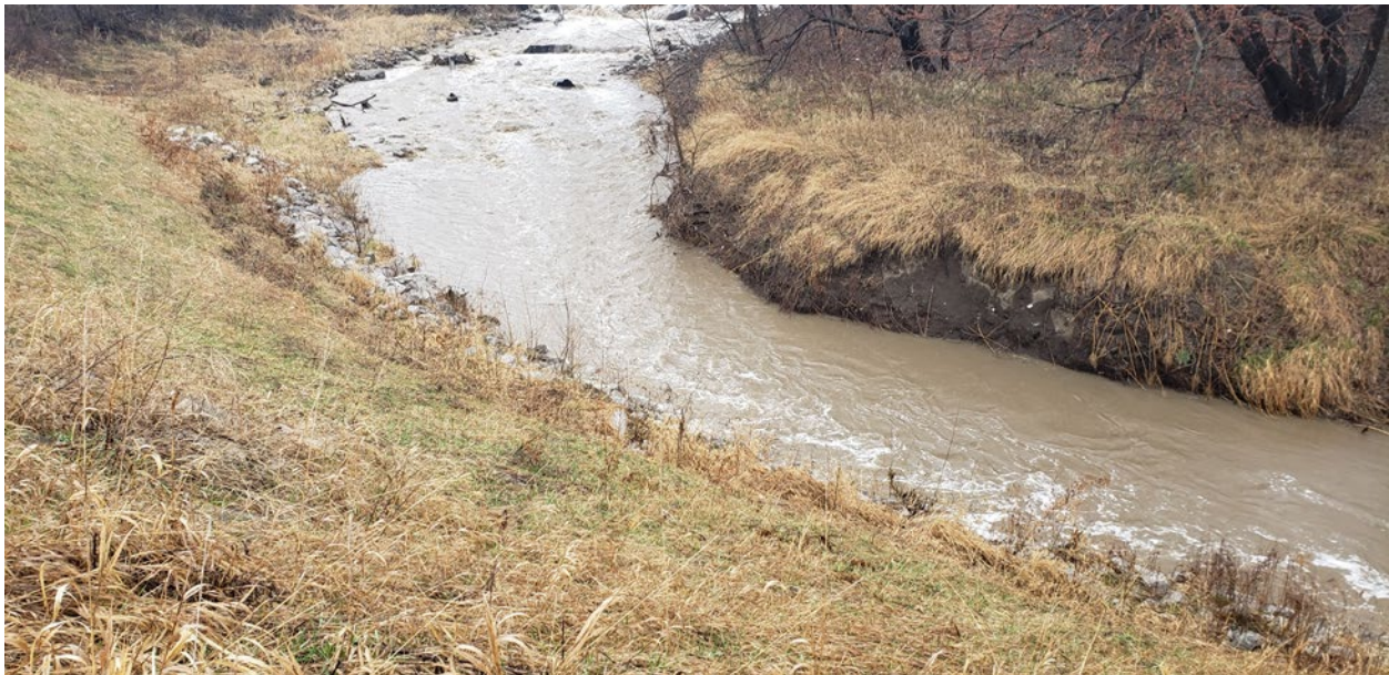
Figure 8-17: EWN LPSTP Project Completed on South Papillion Creek-Reach 3
