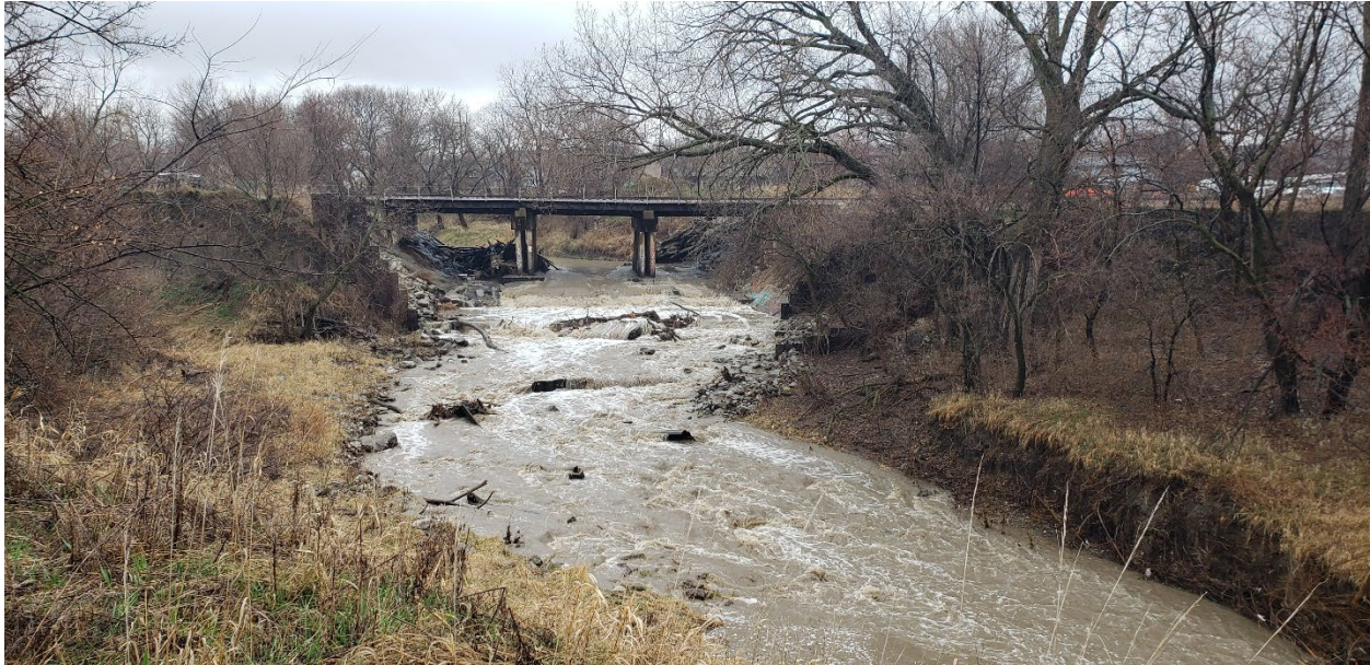
Figure 8-8: FG Reach 3, South Papillion Creek – Illustrating Railroad Bridge GCS
