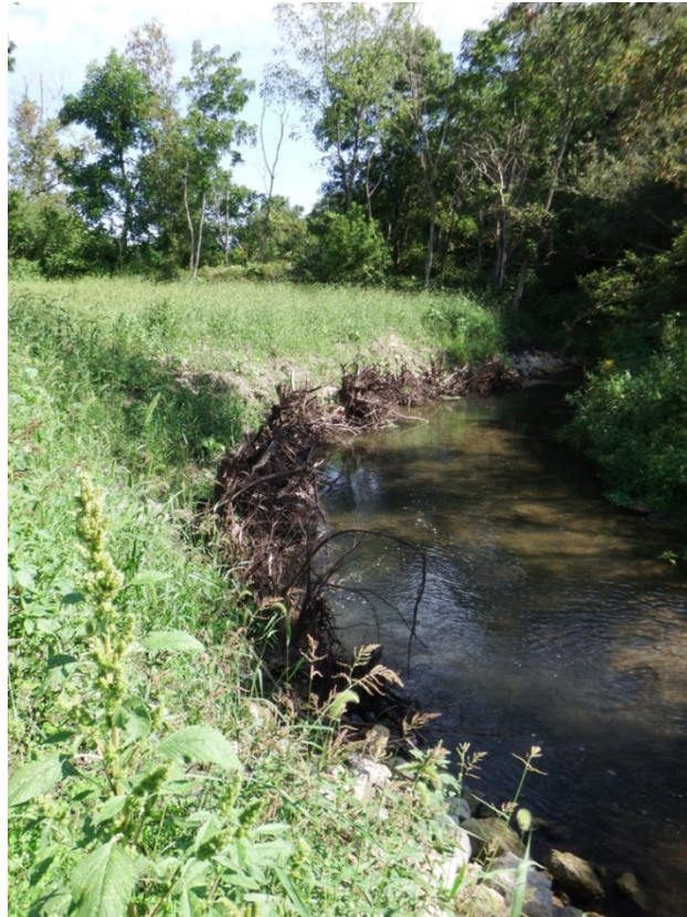
Figure 6-17: Black Walnut Creek LPSTP/Rootwads/Tree Plantings/Prairie Grass
