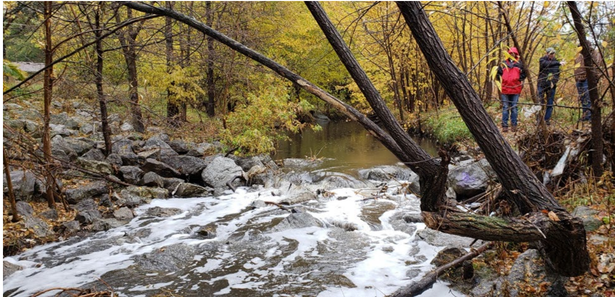
Figure 8-18: Lincoln, NE – Beal Creek Rock Riffle Grade Control Structure
