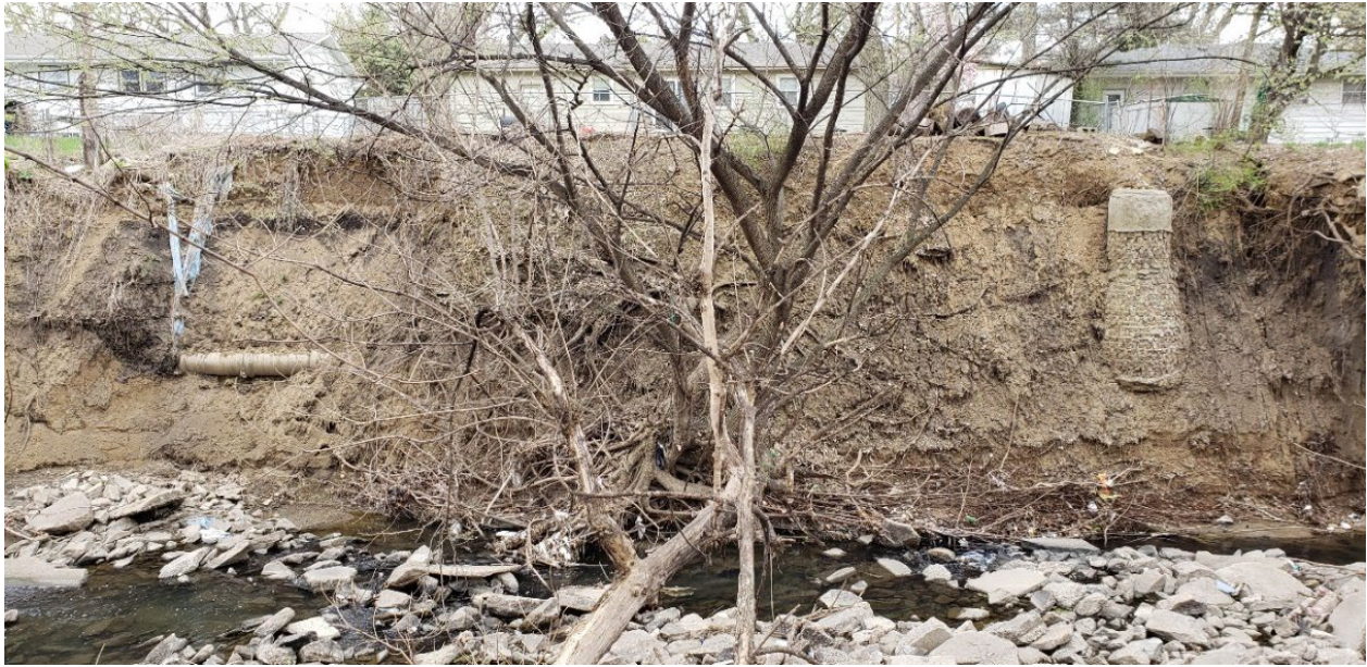
Figure 4-6: Cole Creek Channel and Bankline Showing Riprap Rubble
