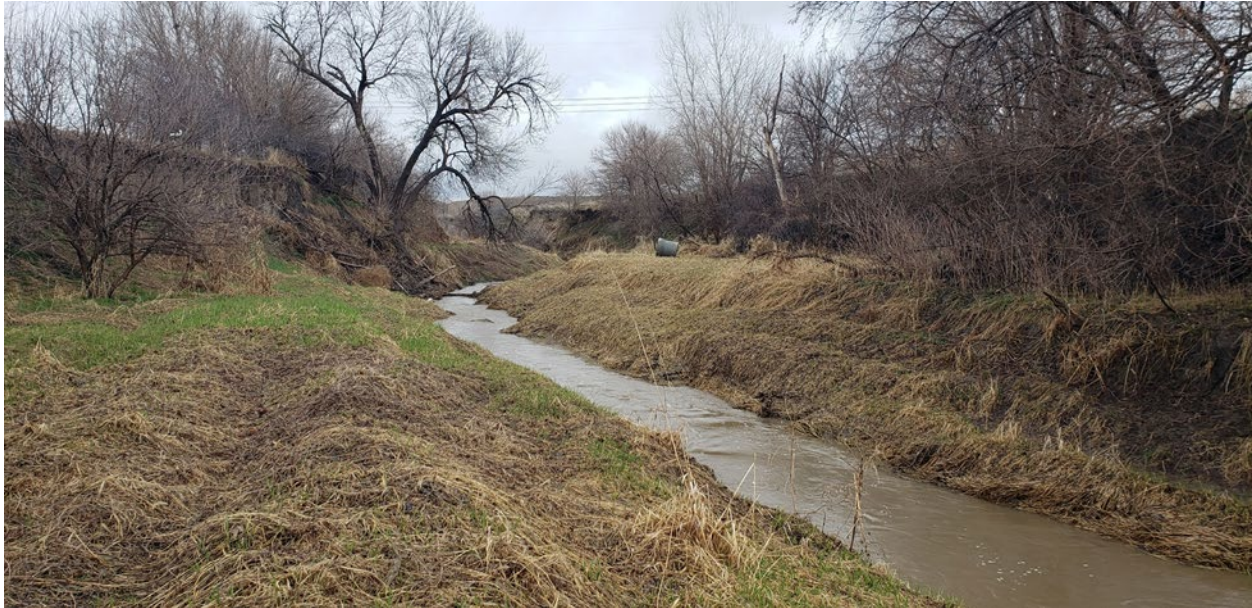
Figure 8-10: FG Reach 6, South Papillion Creek – Upstream of Giles Road Culverts Showing Aggraded, Stable Channel Reach
