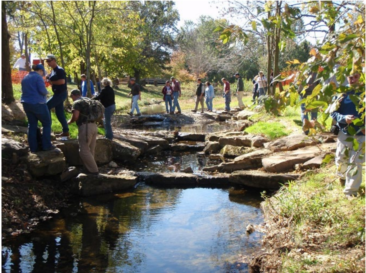
Figure 8-19: Fayetteville, AR, Urban Creek with Cross-Vein Grade Control Structures
