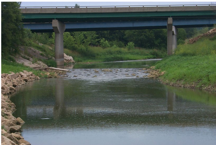
Figure 6-12: Sinsinawa River, IL EWN Loose Rock Riffle Grade Control Project
