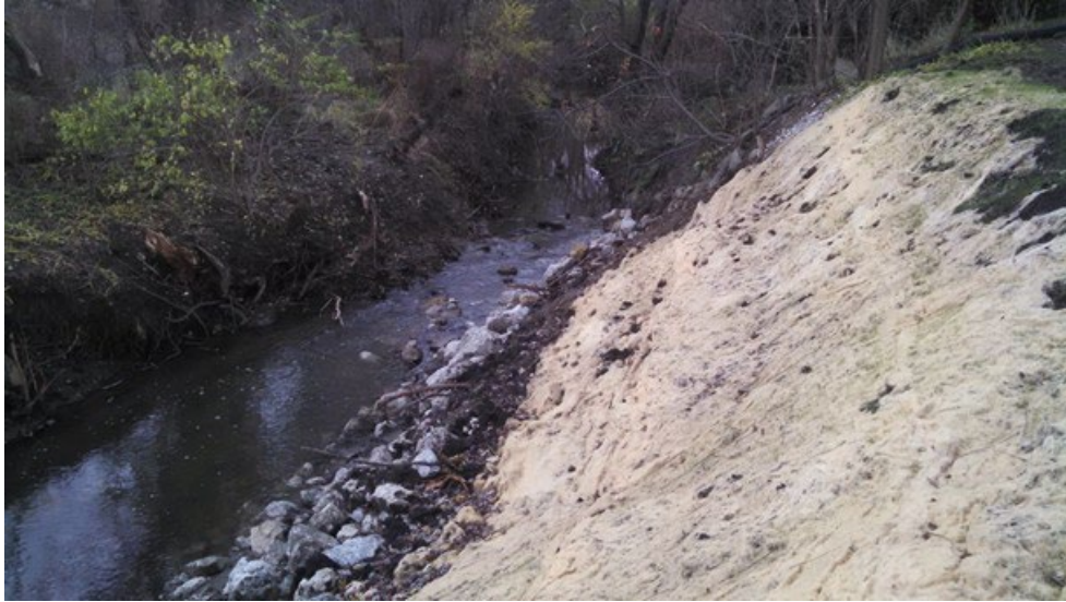
Figure 6-7: EWN LPSTP Project with Erosion Control Matting on Mid- and Upper Banks
