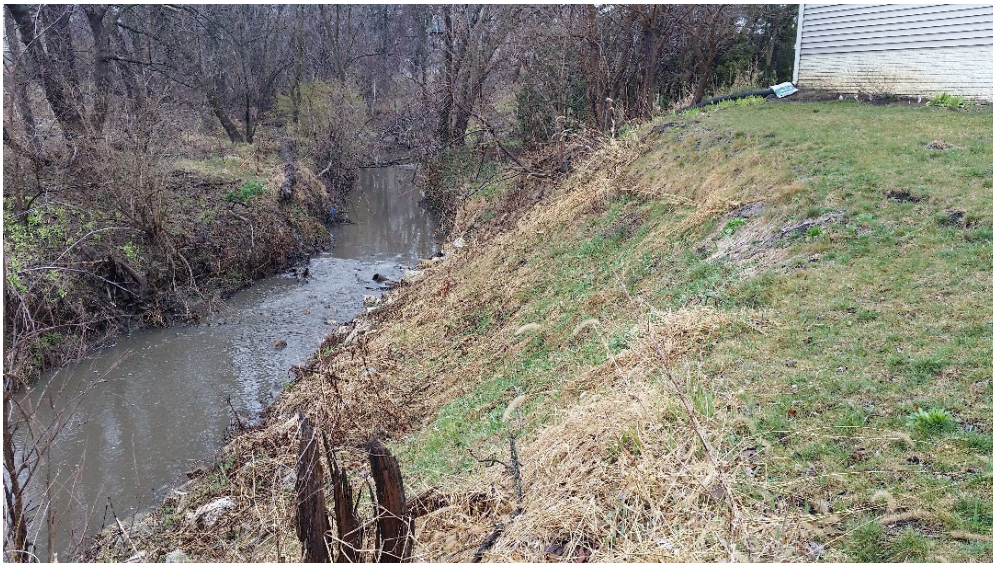
Figure 6-8: EWN LPSTP Project Two Years After Construction
