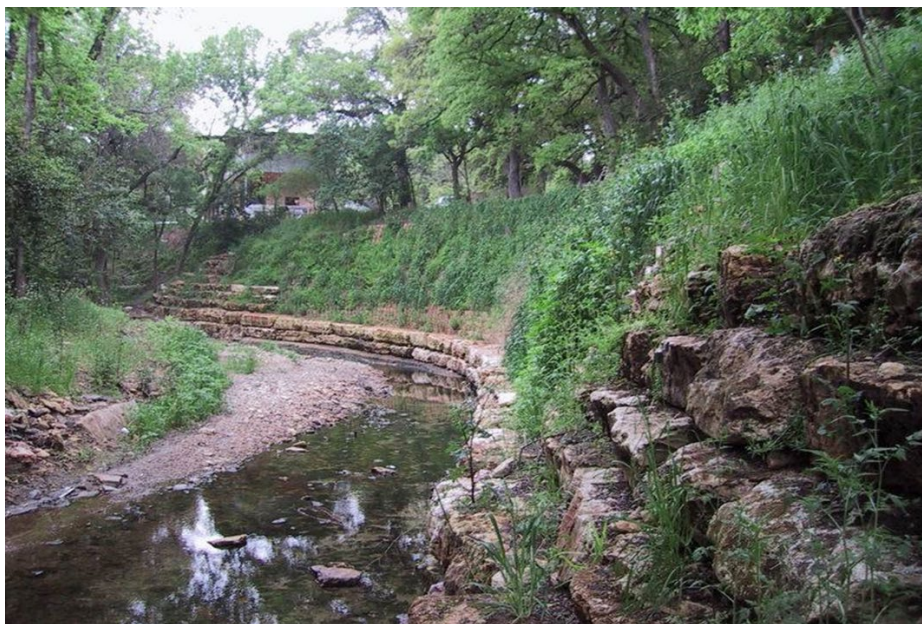
Figure 6-4: Example – Vertical Stabilization Using Landscape Boulders
