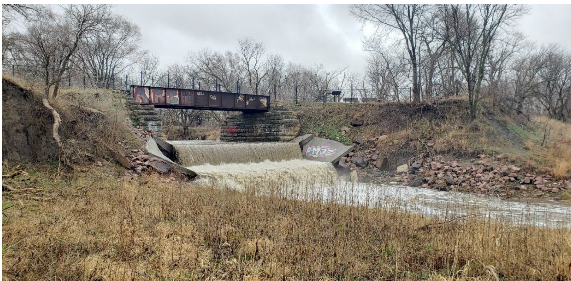
Figure 5-22: Concrete GCS at the Mouth of Hell Creek
