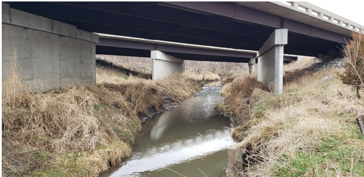
Figure 5-28: Grade Control Structure Located Under Blair High Road Bridge – Thomas Creek
