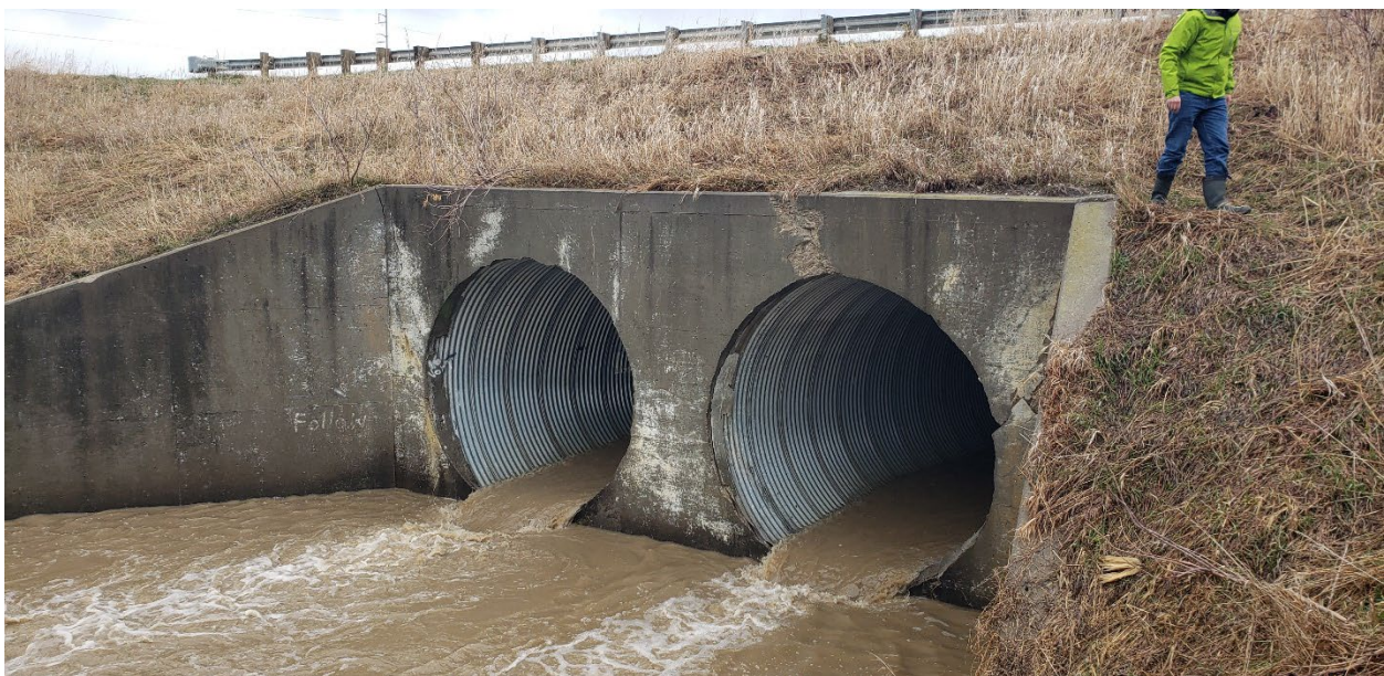
Figure 8-9: FG Reach 6, South Papillion Creek – Giles Road Culverts
