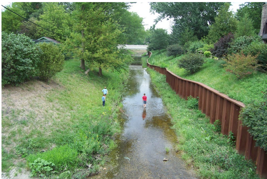
Figure 6-1: Example – Metal Sheet-pile Wall
