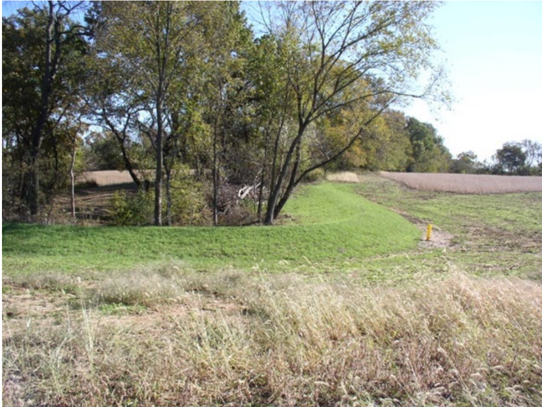
Figure 7-6: Example Water and Sediment Control Basin (WASCOB)
